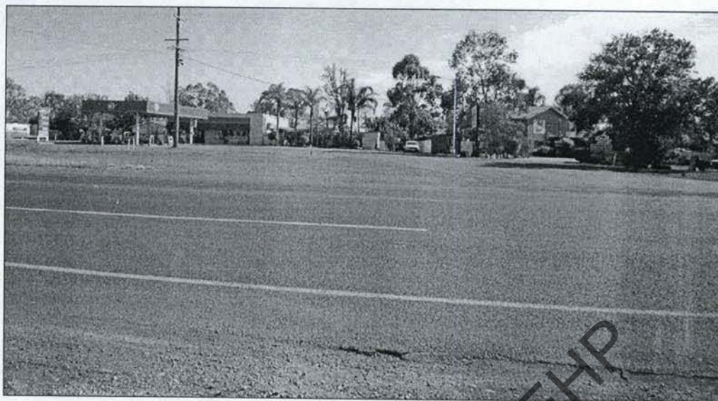
Plate 3: Warrego Highway looking at the east entrance of the access loop road
