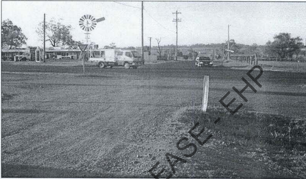
Plate 1: Steger Rd facing south towards the intersection of Warrego Hwy/O'Mara Rd/Steger Rd
