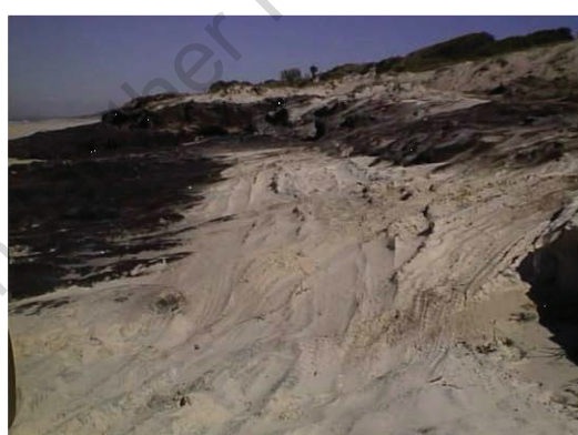
Photo 2 vehicle entry for illegal bypass track
