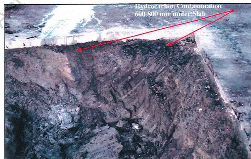
Photo 4A- Pit 1 excavation looking east
