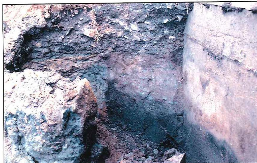
Photo 2A- Hydrocarbon contamination adjacent to rat wall BH-6
