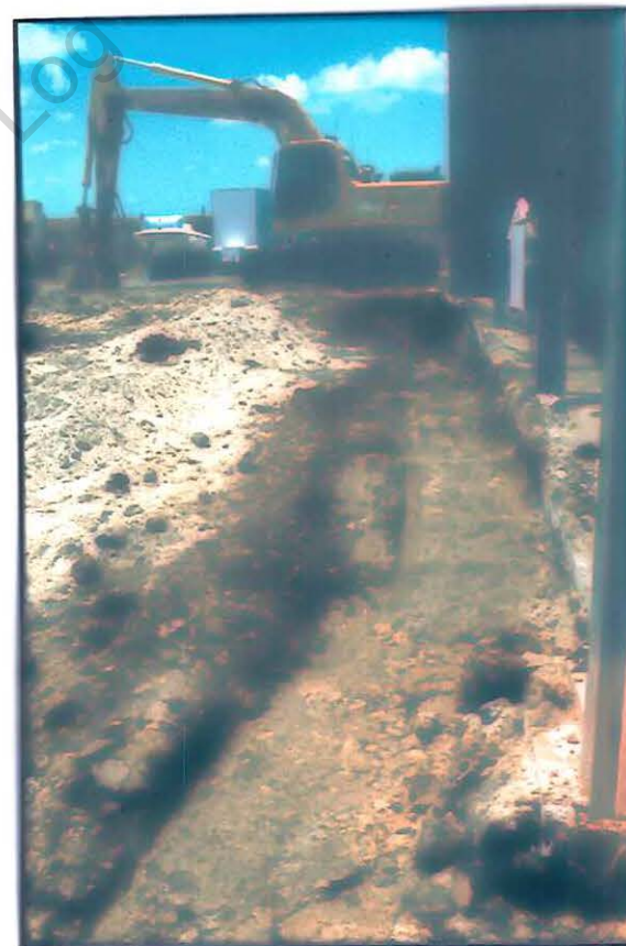
Photo 3B- Construction of clay barrier northern side of shed.
