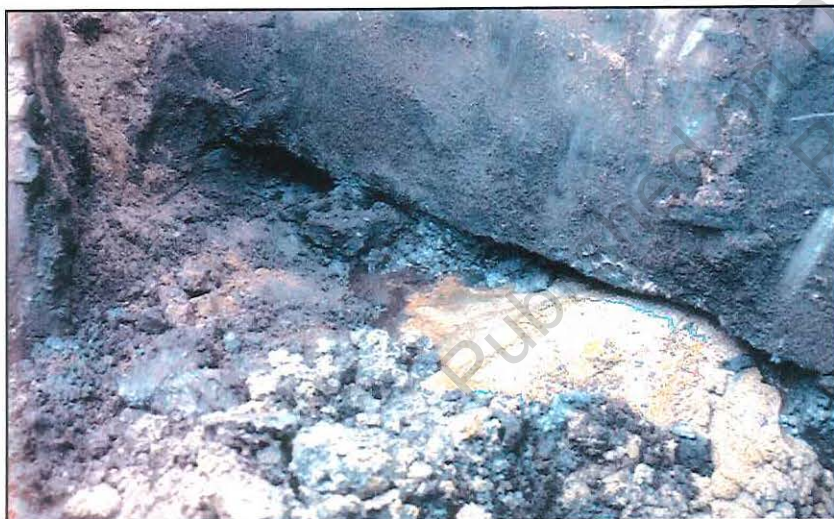
Photo 3A- Hydrocarbon contamination flowing from beneath rat wall BH-6
