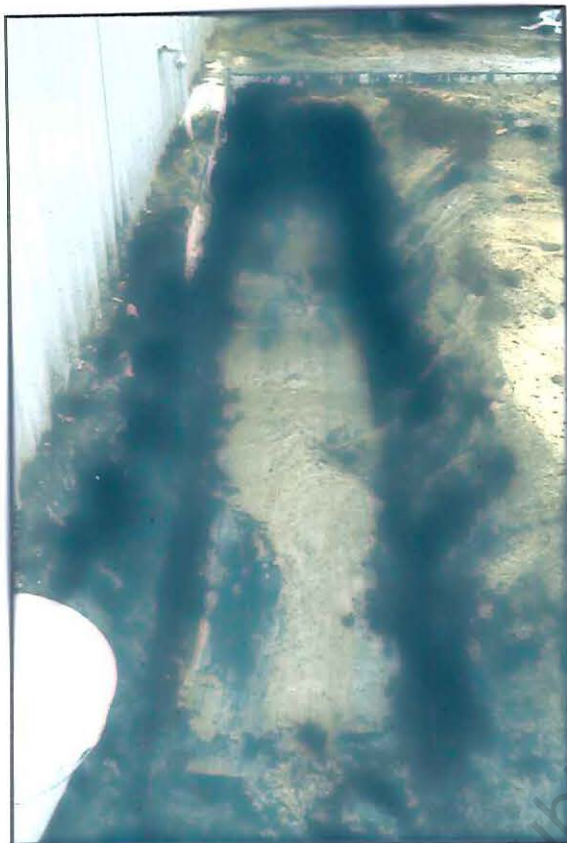
Photo 1B- Construction of clay barrier western side of shed.
