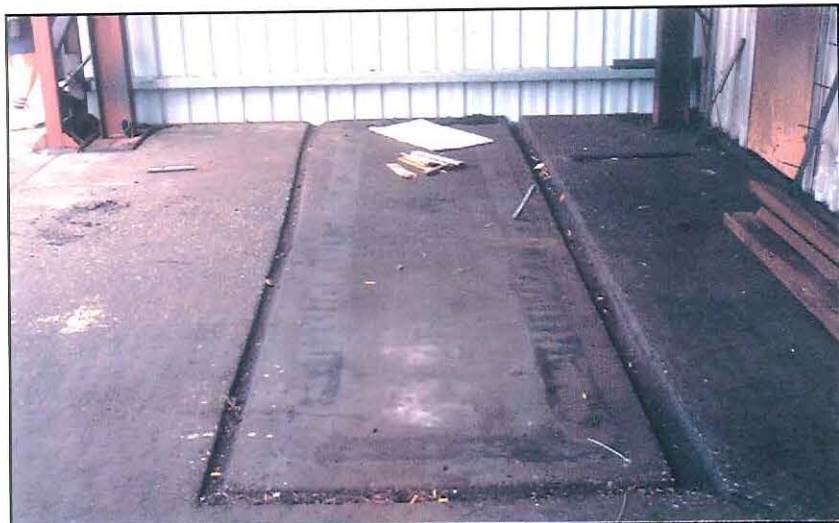
Photo 1A- Lubrication bay adjacent to BH-6
