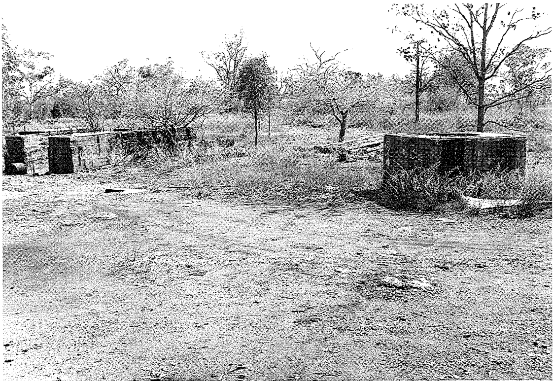
Boiler and engine house mounts, with chimney concrete base on right. Looking SW.
