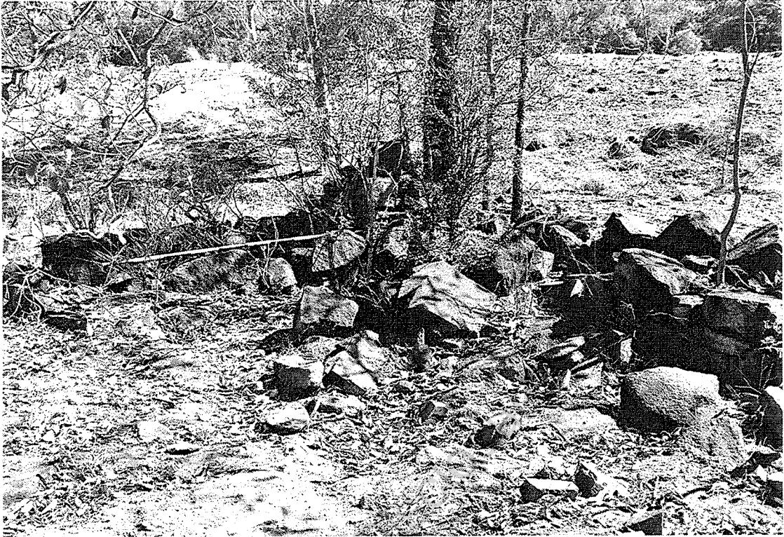
Eastern battery site: collapsed stonework of boiler mount, looking N. (Refer to plan)
