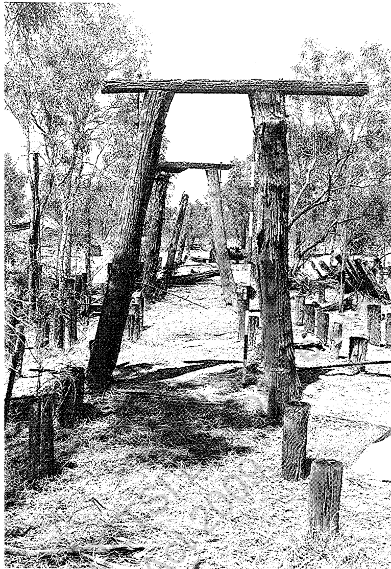
Cyanide vat timber stump mounts on tailings. Looking S.
