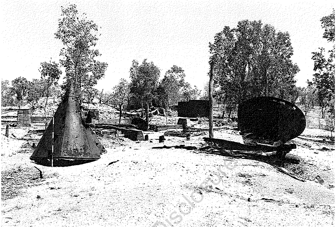
General view of battery site with Babcock boiler house in background. Looking W.
