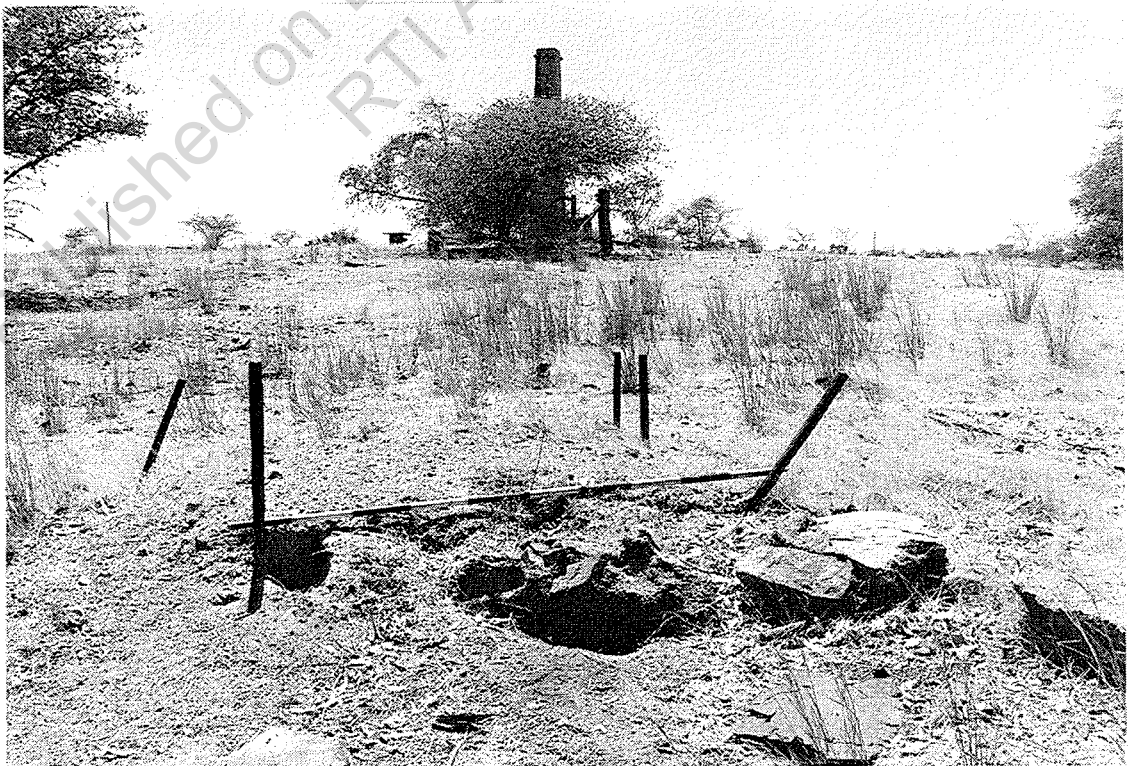
Five head stamp battery foundations, looking NW.
