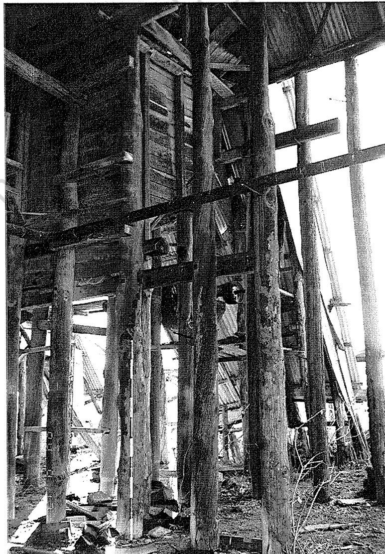
Elevated timber ore bins, looking W.
