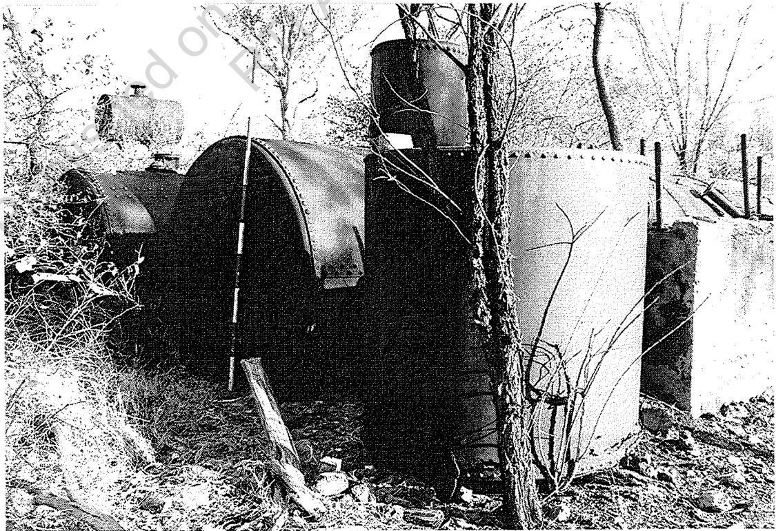
Battery boiler house site, looking NW.
