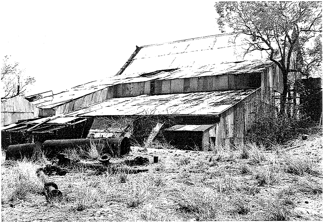
Rear of battery shed, looking W.
