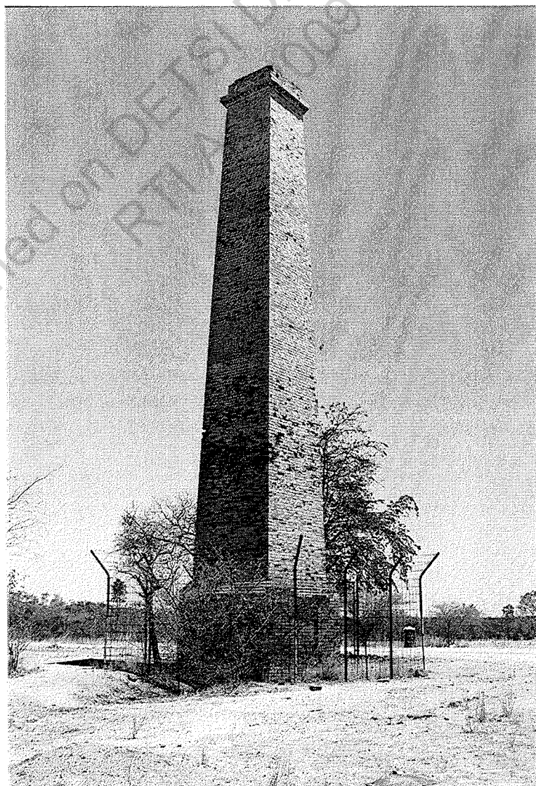
Brick chimney, looking SW.
