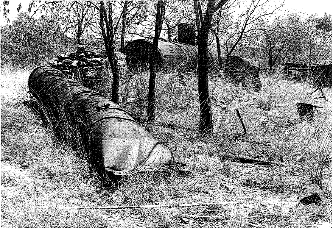
Fallen stack section with chimney base and Cornish boiler in the background. Looking W.
