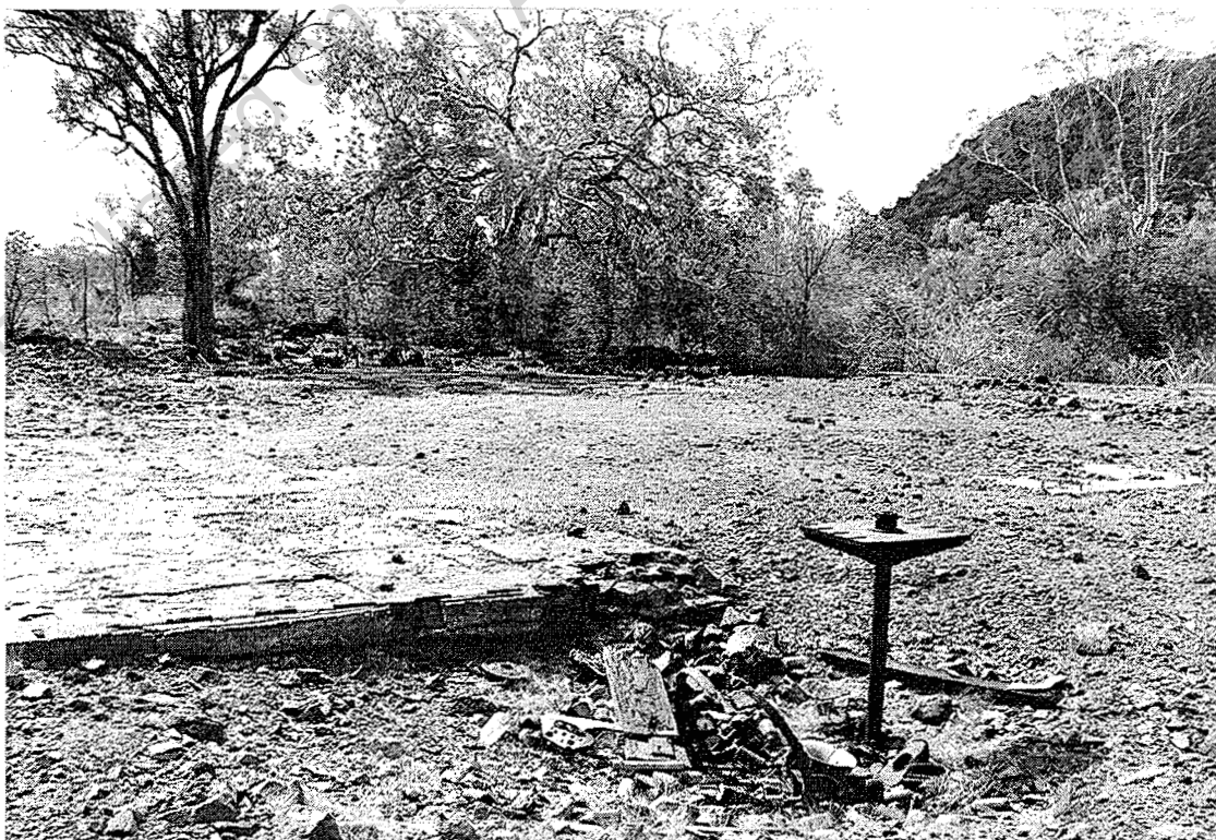
Smelter site showing blast furnace column, slag dump (right) and slag floor (left). Looking NW.
