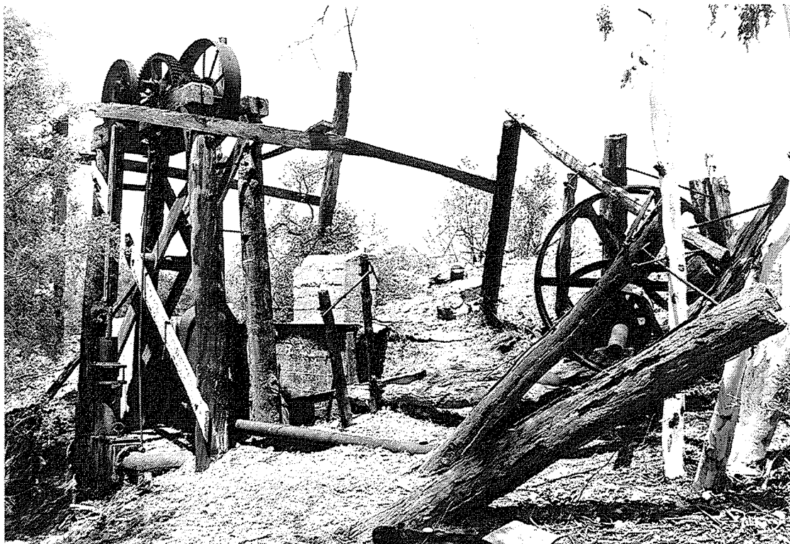
2 cyl. ram pump on the bank of the Copperfield River. Looking S.
