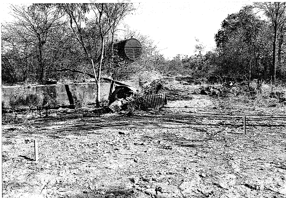
Battery shed foundations (left) and boiler house site (centre). Looking S. Survey pegs for new bridge approach in foreground.
