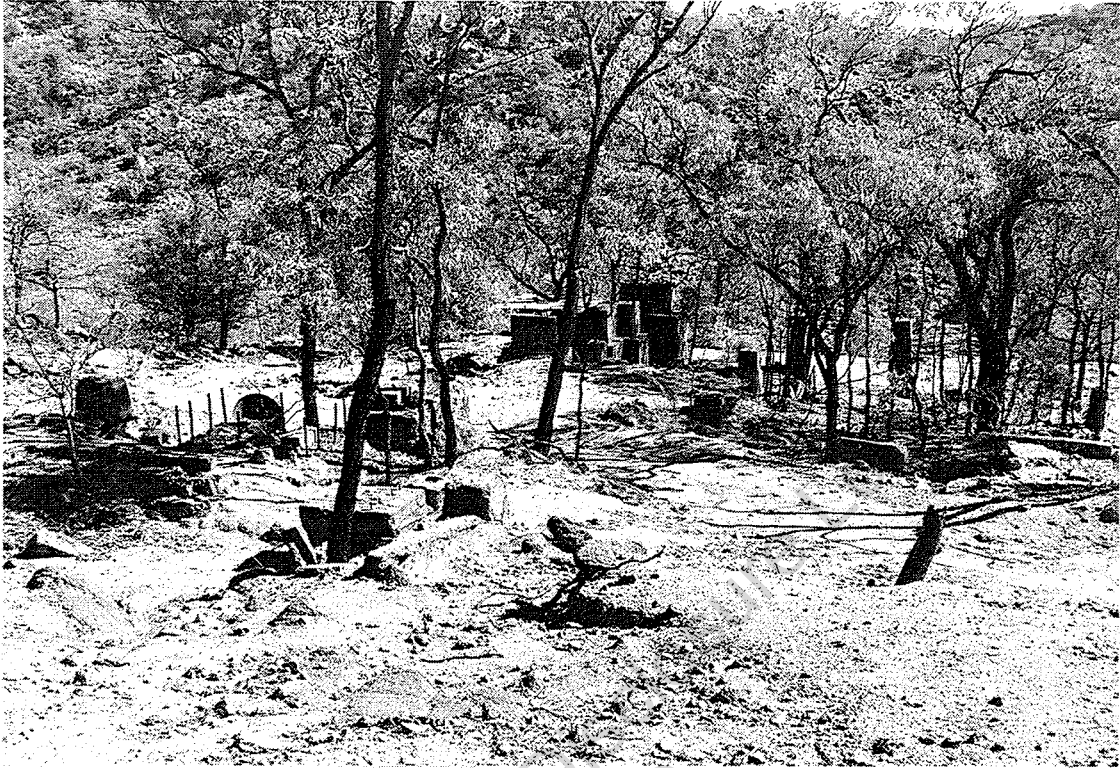
Battery concrete foundations and mounts looking S.
