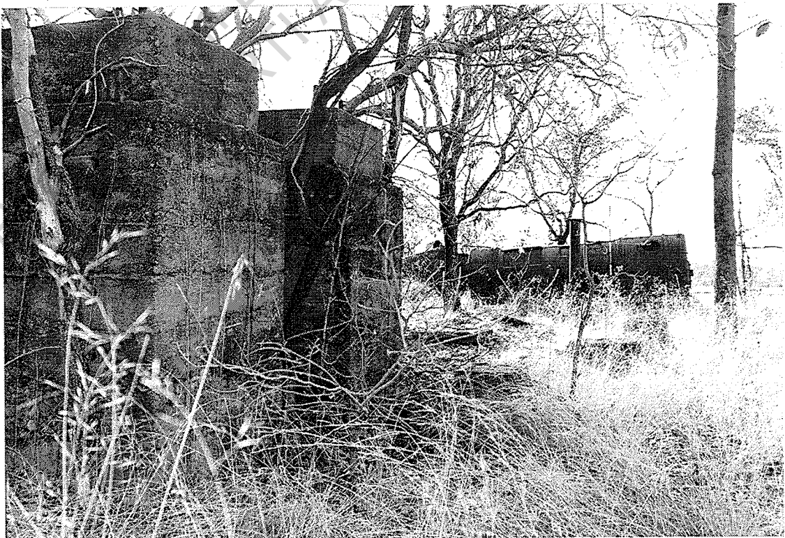
2m high concrete mount (air compressor ?), with portable engine in background. Looking NW.
