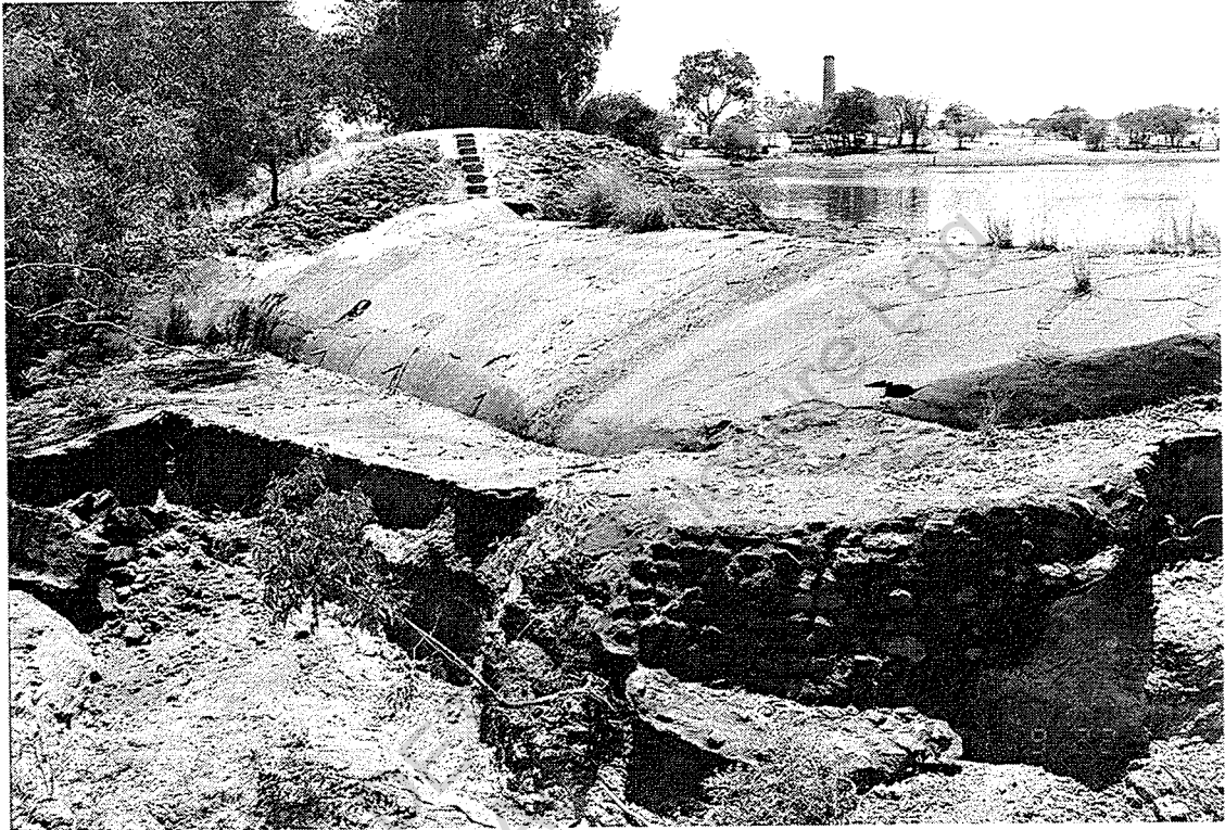
Dam spillway looking NW. to chimney.
