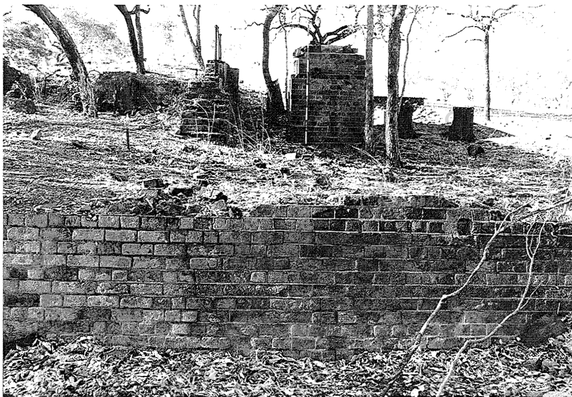
Castleton battery, with boiler and engine house brick mounts in background.
