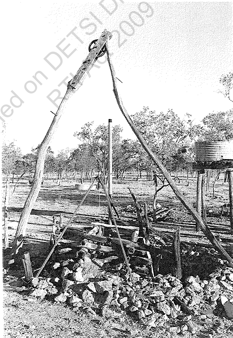
Battery shaft showing bush timber 'whip' hoist.
