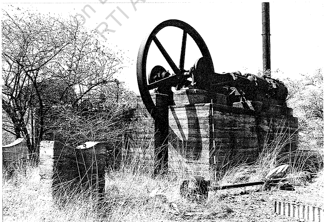
Thompson air compressor on 2m high concrete mount, looking NE.
