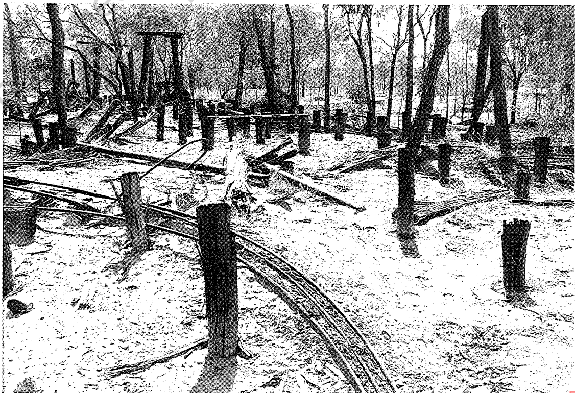
Cyanide plant site showing iron hoops from timber vats (foreground). Looking NE.
