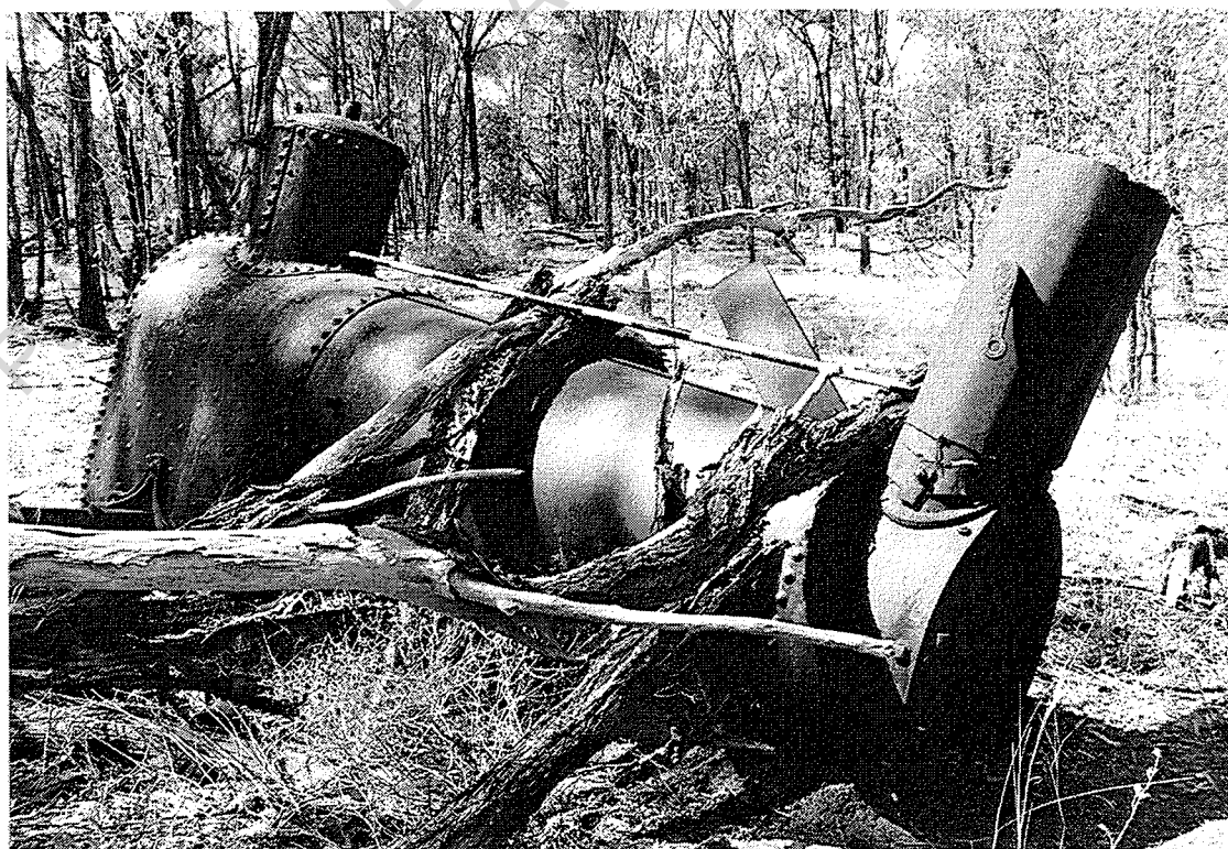
Wet-bottom portable boiler, looking SE.
