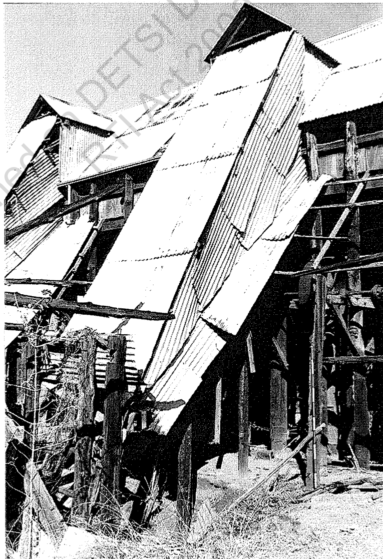
Battery shed ore elevator housing, looking E.
