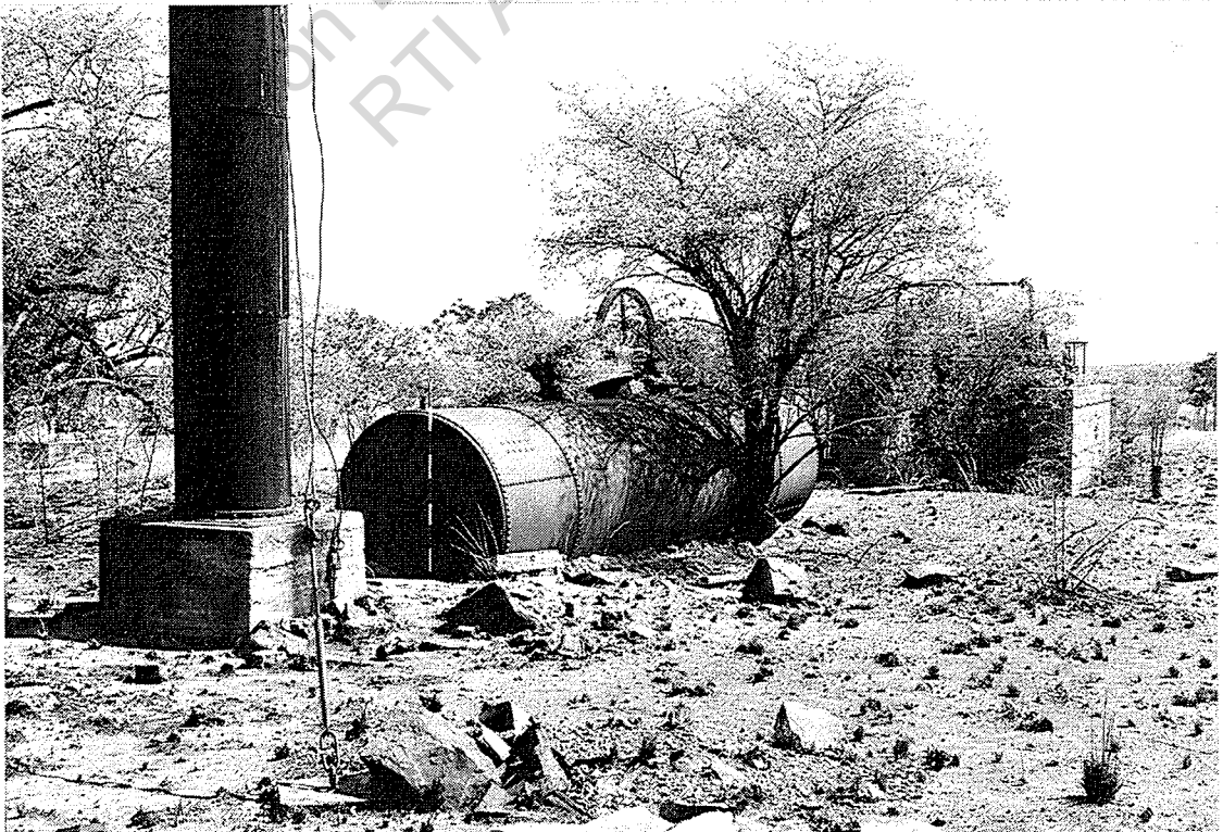
Winding engine plant (foreground), with Cornish boiler and stack. Looking E.
