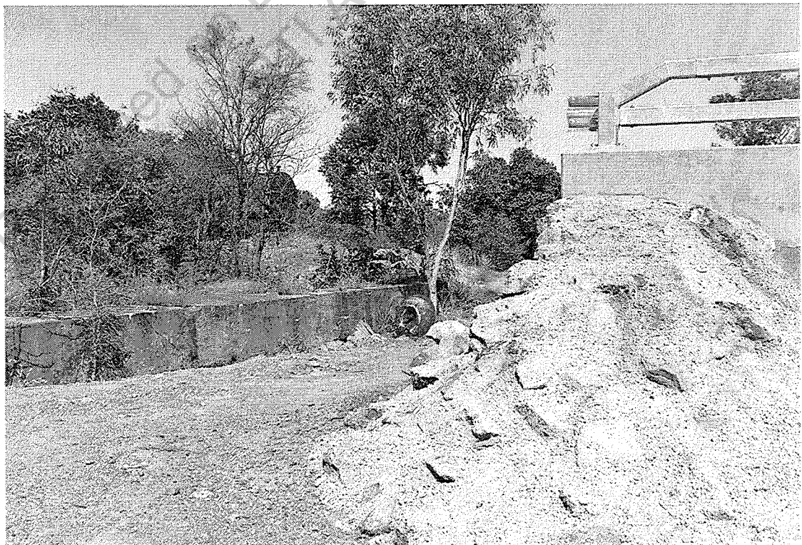
Enterprise Battery with new bridgeworks (June 1995). Boiler visible in background at right. Looking SE.
