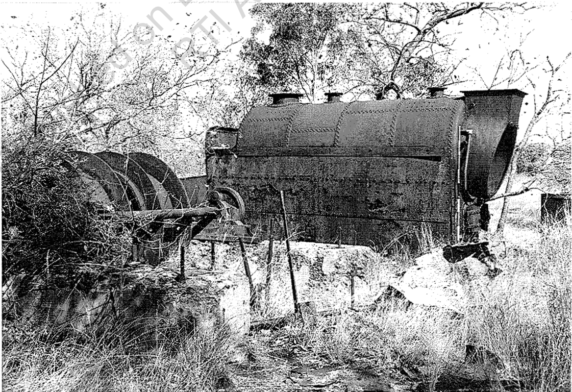
Stuart & McKenzie winding engine and colonial boiler, looking SE.
