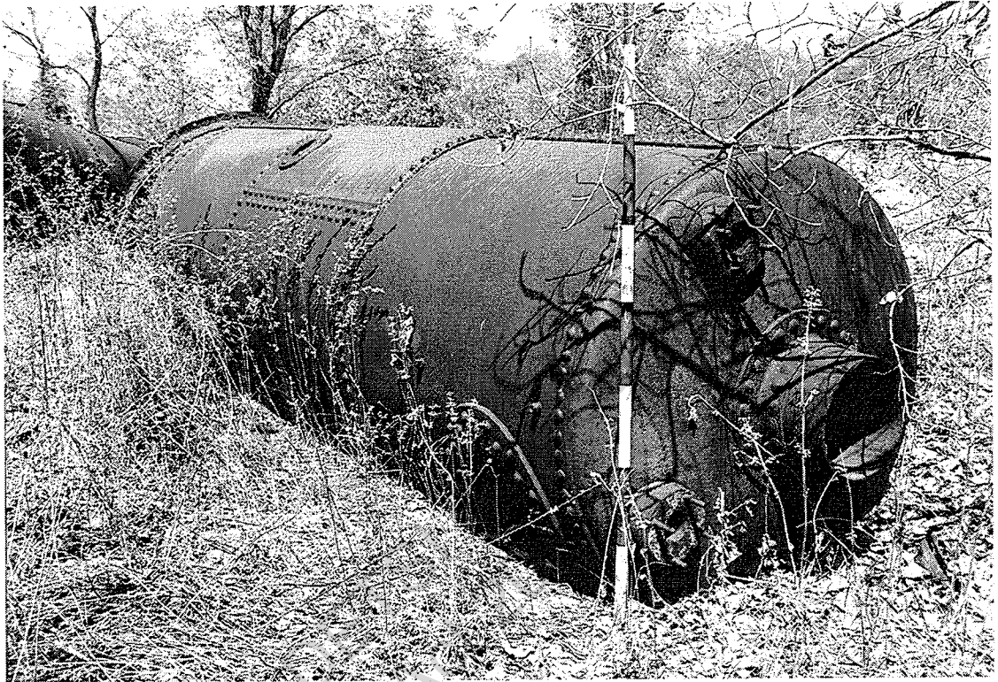
Vertical boiler (n/i), looking S.
