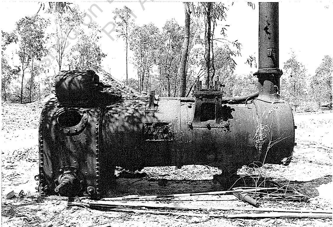
Cyanide plant Clayton & Shuttleworth portable engine, looking S.
