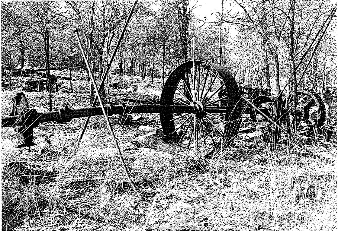
Battery site, looking S. with fallen belt wheel shaft in foreground.
