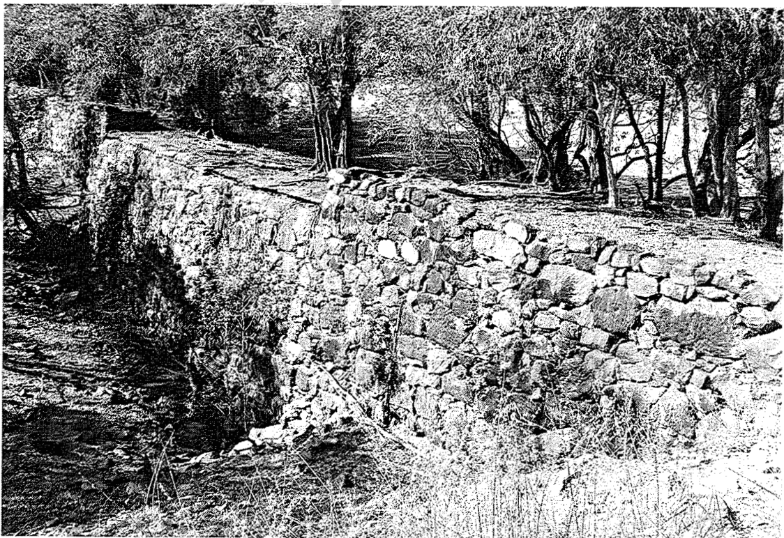
Overshot weir showing spillway. Looking N.
