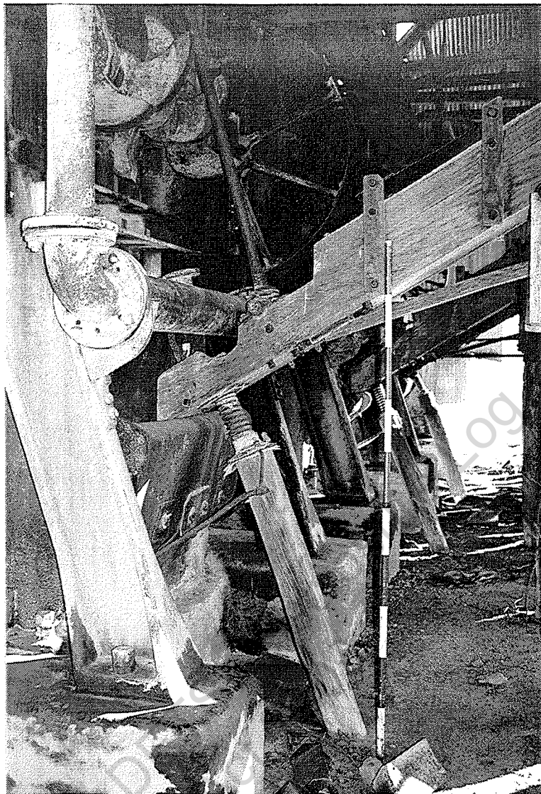
Feed from ore bins to mortar boxes, looking SW.
