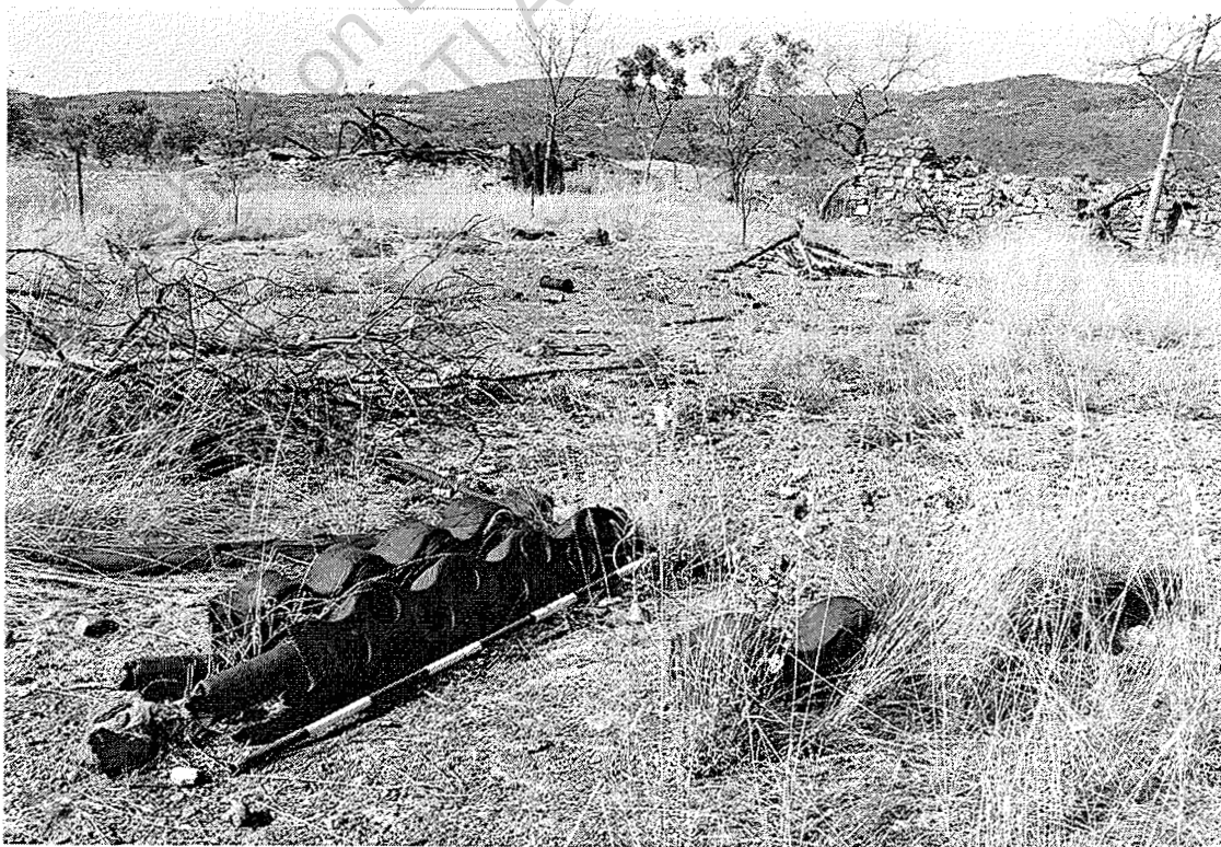
Tramway stage (background left) with B & W boiler tube ends (foreground).
