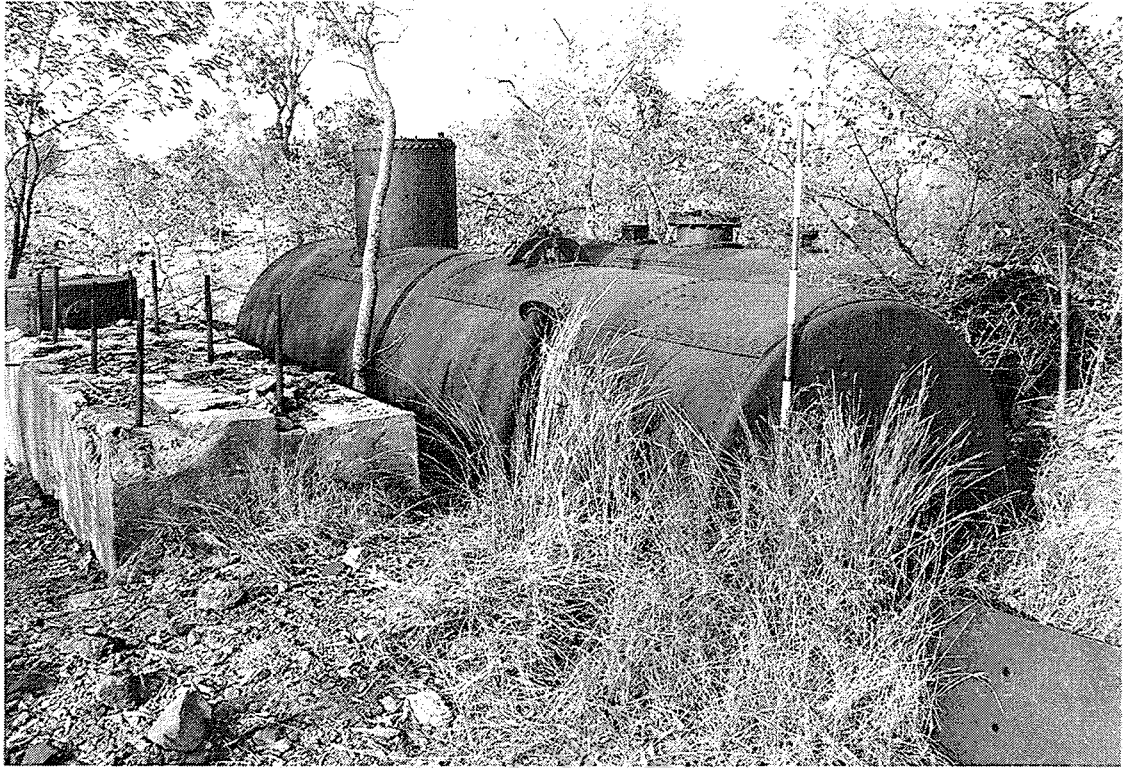
Battery boiler and engine house site, showing Langlands Cornish boiler (centre). Looking SW.
