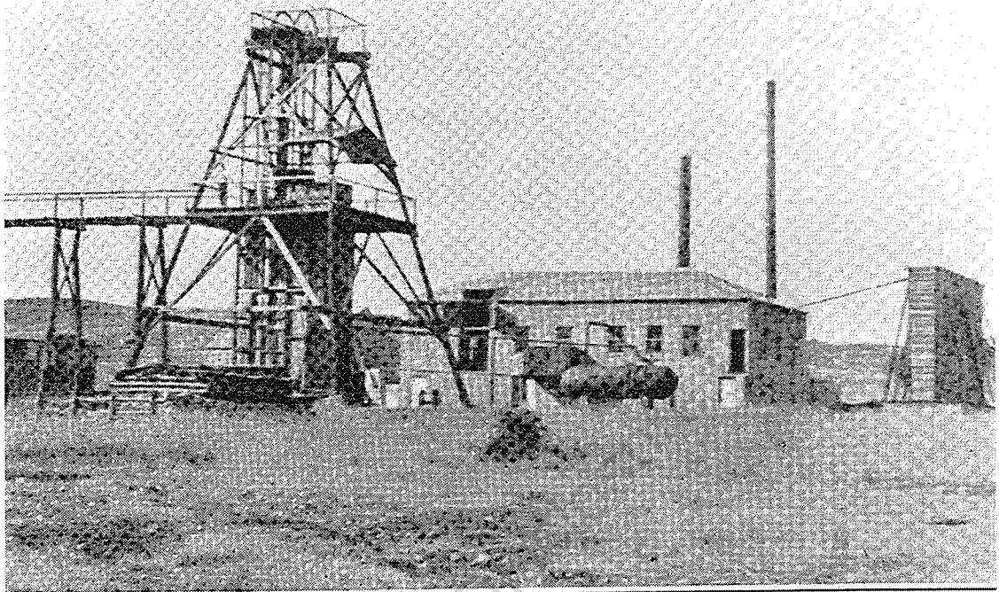
Main shaft headframe and winding engine shed. Looking E. Q.G.M.J. 15 August 1917, p.391.
