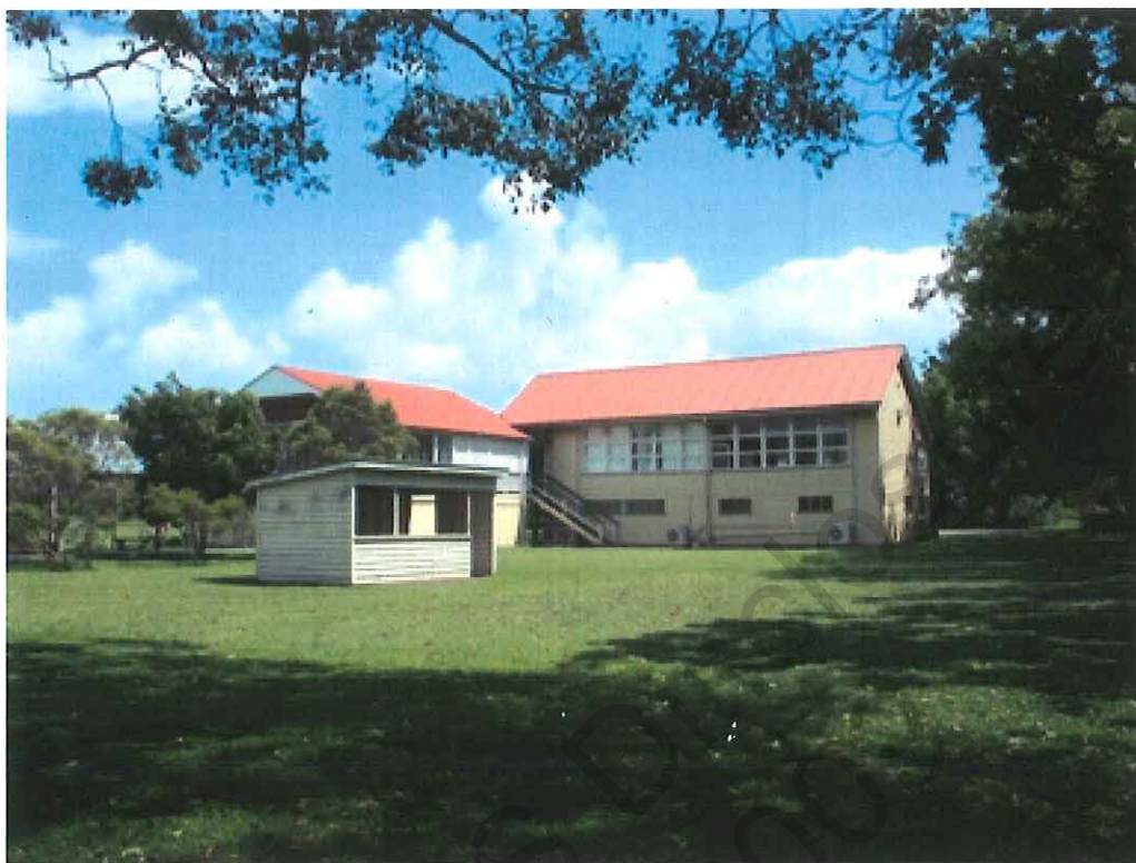
Figure 10: View from south L – R : 1913 addition, 1956 extensions and alterations on RHS of 1895 addition, tennis shed in foreground with remains of 1929 tennis court
