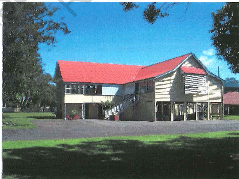
SCHOOL FROM EAST
