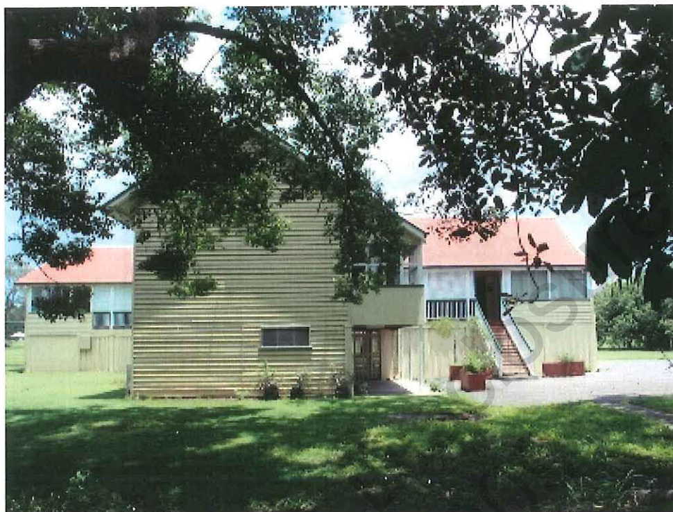
Fig 6: View from Eagle Farm Road, with 1913 building in foreground, original Suter building on RHS and 1895 building on LHS.
