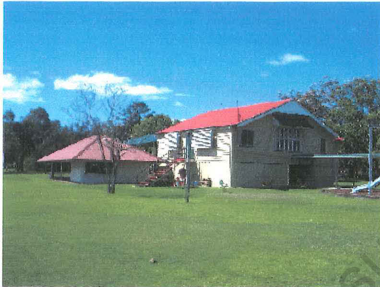
SCHOOL FROM THE WEST
