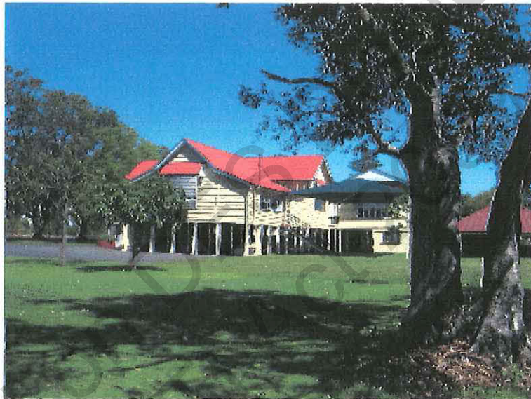
SCHOOL FROM THE NORTH EAST
