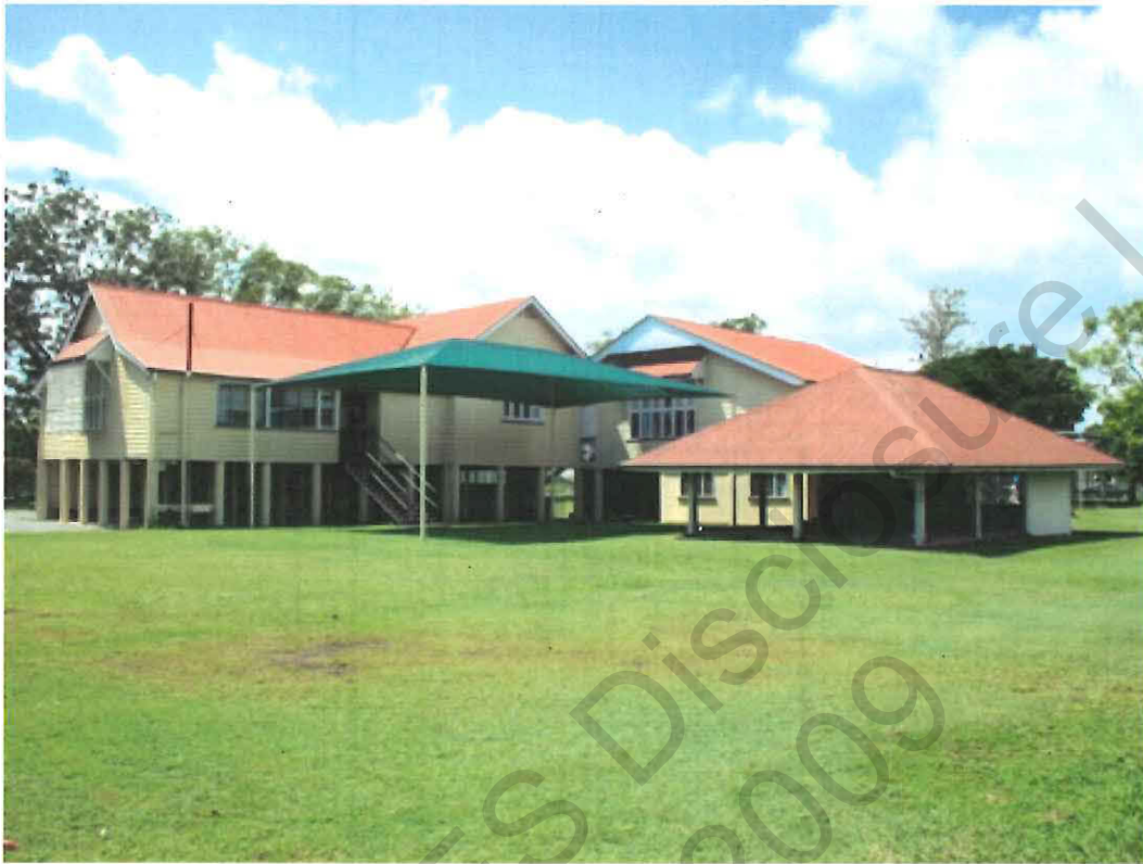
Figure 4: L-R: 1875 structure, 1895 extension, 1913 addition, 1897 play shed
