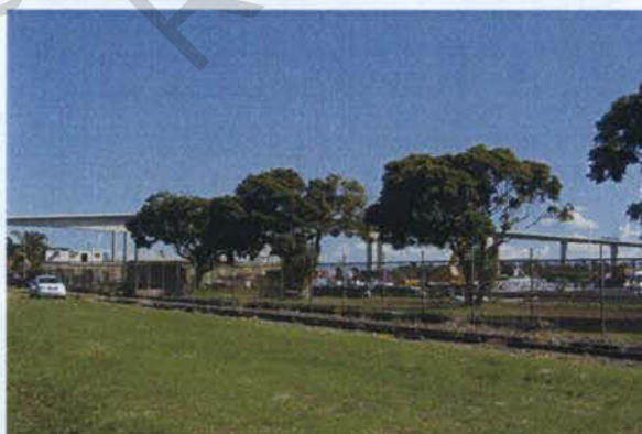
Figure 12: Boat and barge industry northwest of the site
