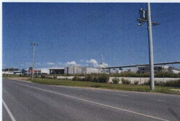
Figure 10: Industry under construction west of the site on Queensport Road
