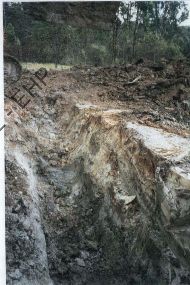
Photograph 4: Excavation of Cattle Dip (viewed towards north east)
