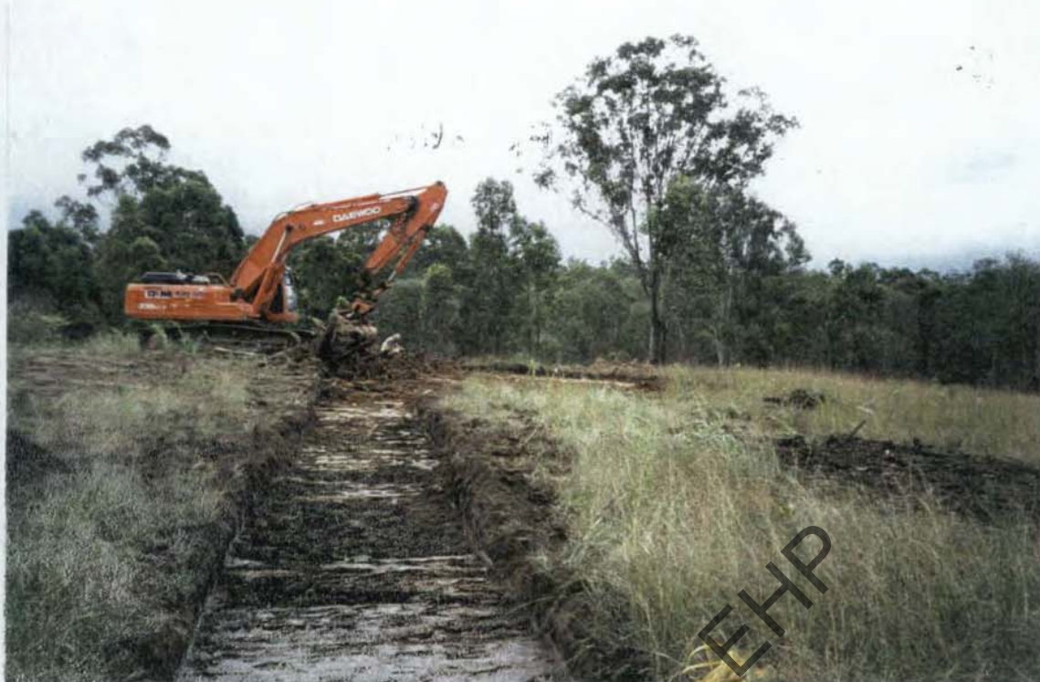
Photograph 1: General View of Excavation (viewed towards north east)
