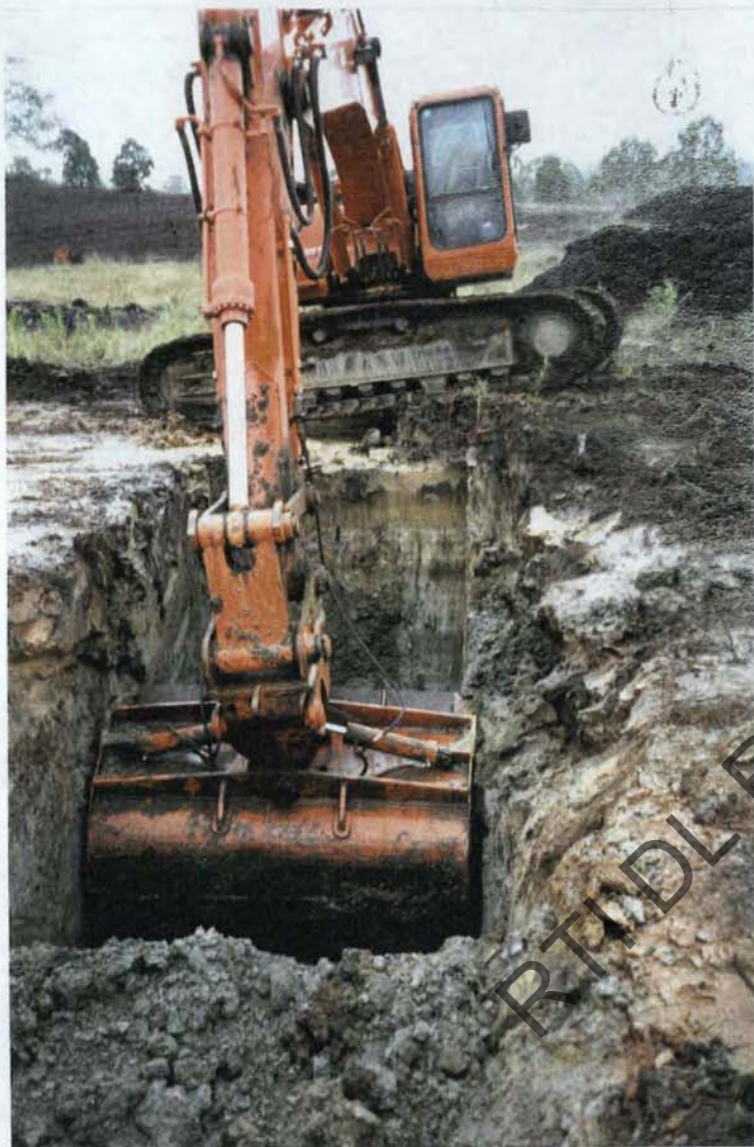
Photograph 3: Excavation of Cattle Dip (viewed towards south west)
