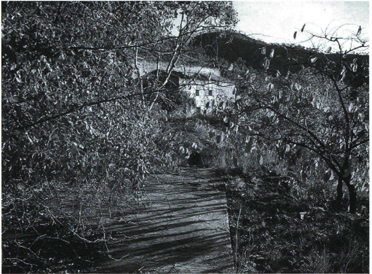
A long concrete slab on the side of a hill with the 3FSHQ in the background in June 2003.
