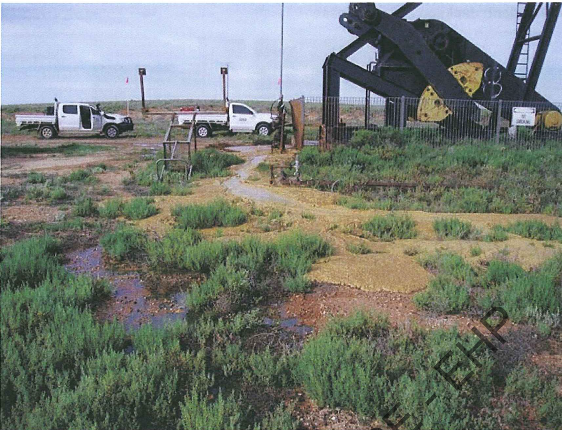
Jackson #38. Showing extent of soil contamination.
