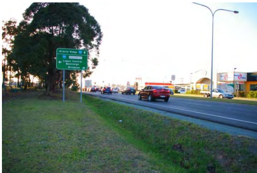
Compton rd access location, viewing west
