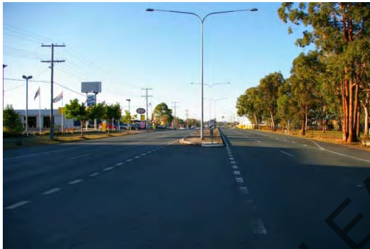
Kingston Rd median break, viewing north
