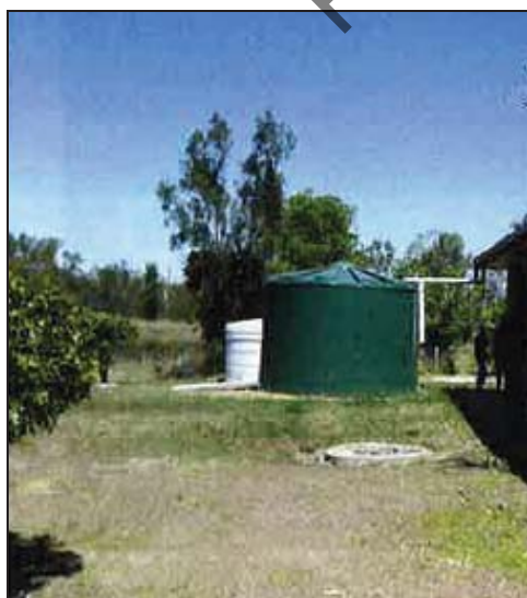
Figure 2. Polyethylene Tank, with White Tank behind.
