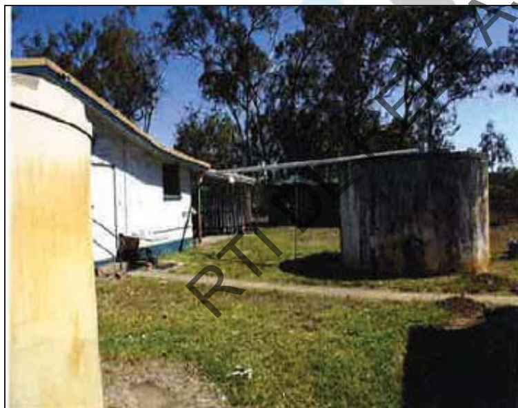
Figure 6. Polyethylene (left hand side) and Concrete tanks, where
