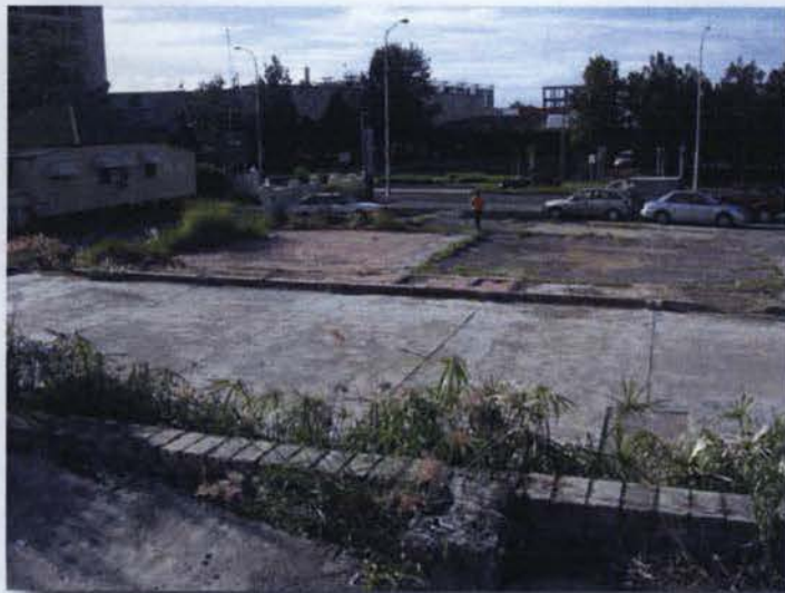
Photo 1 - Initial layout of site during Stage 1 and 2 works, view to the south showing the hardstand areas.
