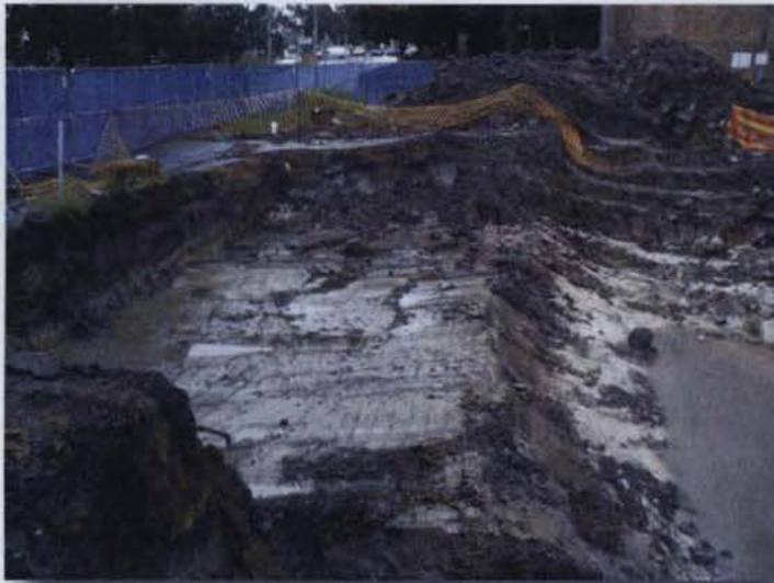
Photo 4 - UST Excavation, on Vulture Street boundary looking west.
