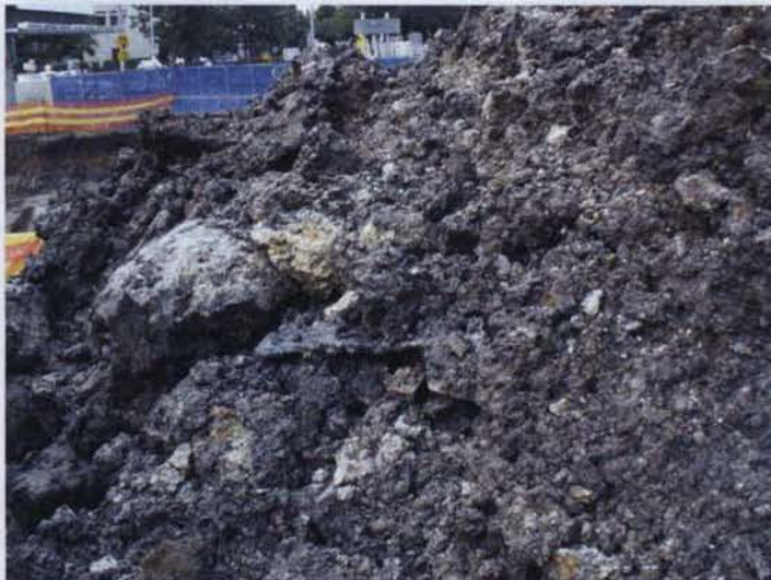
Photo 7 - Stockpile material from UST Excavation.
