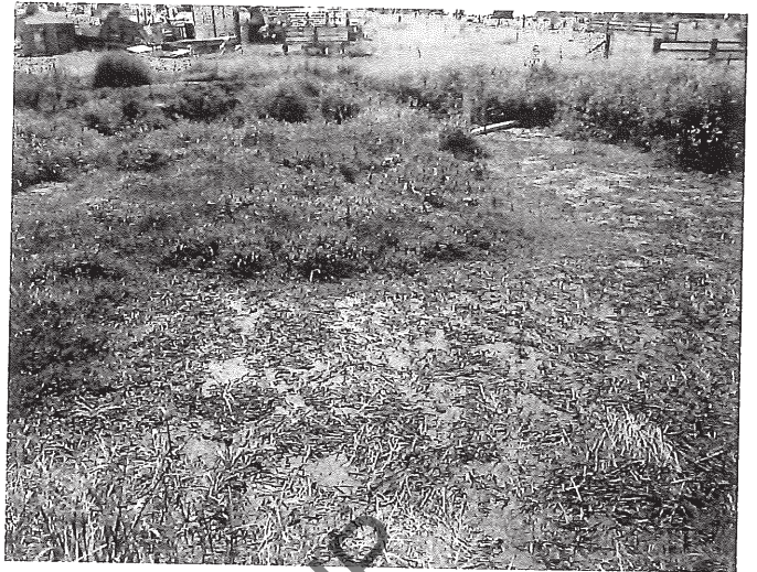
Photo 2: 3 rd Anaerobic Pond
