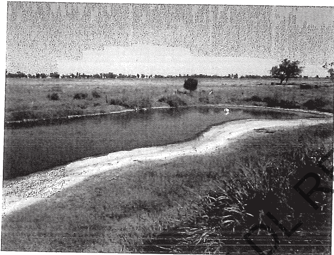
Photo 3: Wet weather storage dam
