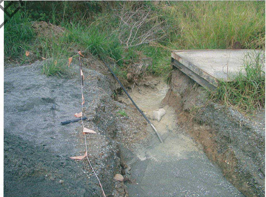
Photo 4: Wastewater flowing into the sediment system on the southern boundary.
