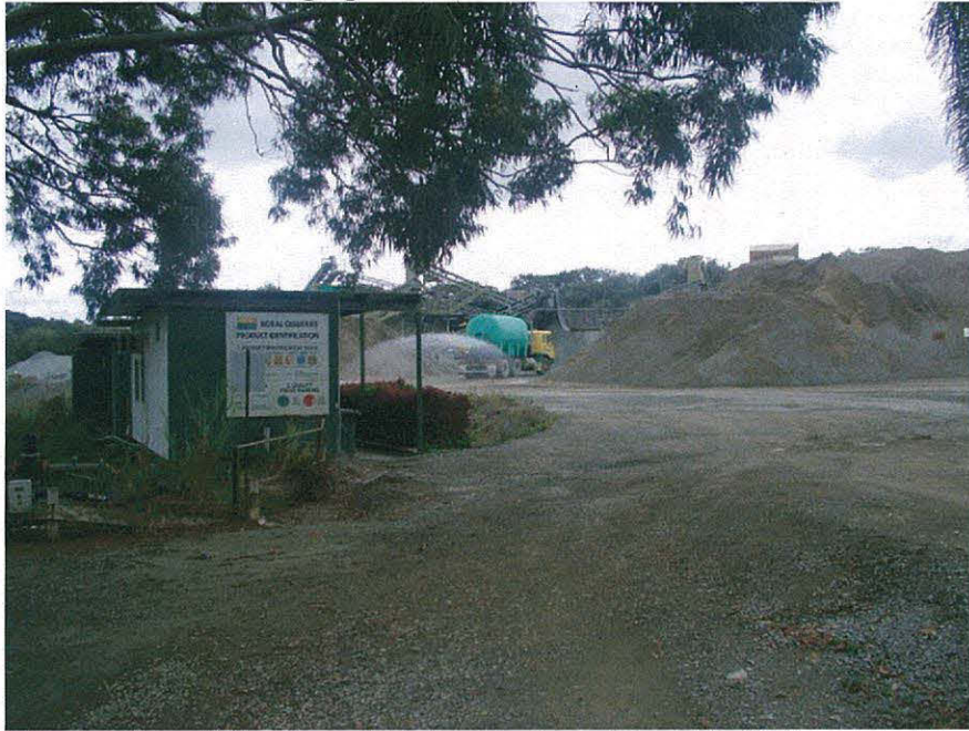
Photo 1: Shows the water truck and new green tank on the back.
