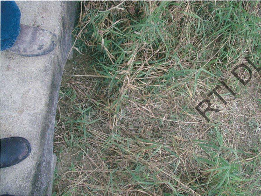
Photo 6: Outlet from the culvert under the road. Water then flows into a cane paddock (photo 7).
