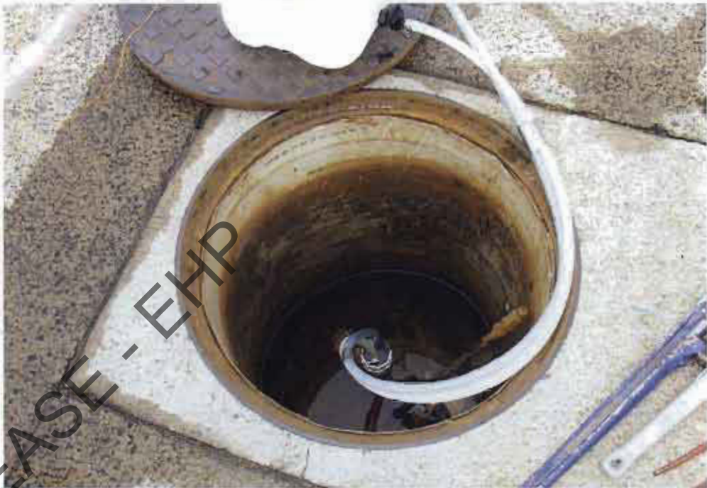
Inside MPE oil & air sparger
