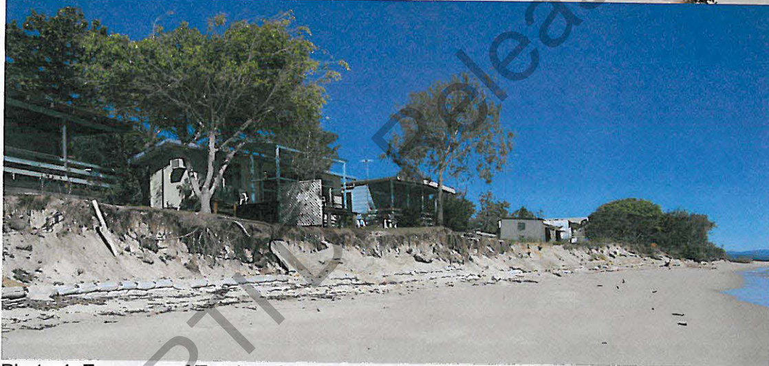
Photo 4: Exposure of Tourism Centre buildings on the edge of the erosion scarp. Note the extensive sand bagging.
