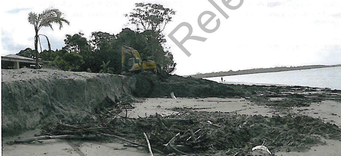
Photo 7: Scraping sand from the intertidal zone at Toogum to reinforce the eroded dune. The sand only persisted for a few weeks and was moved back down the beach slope by a storm event.
