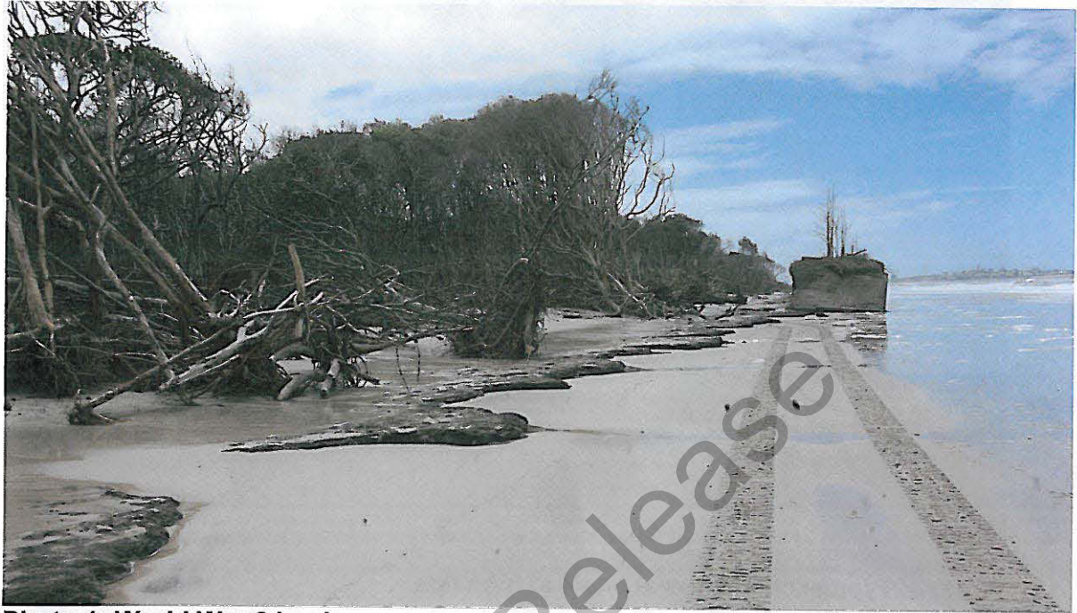
Photo 1: World War 2 bunkers exposed by sea erosion with shoreline retreat into tea-tree swamps.
