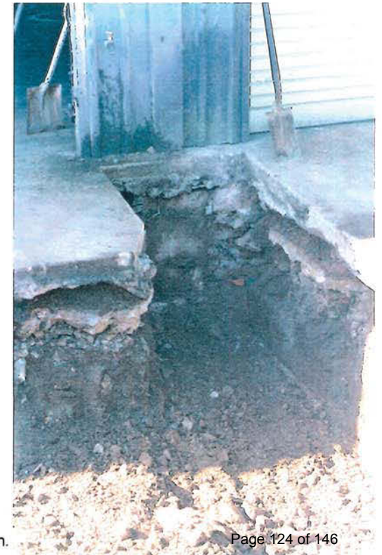
Further excavation of the pump drain area in progress.
