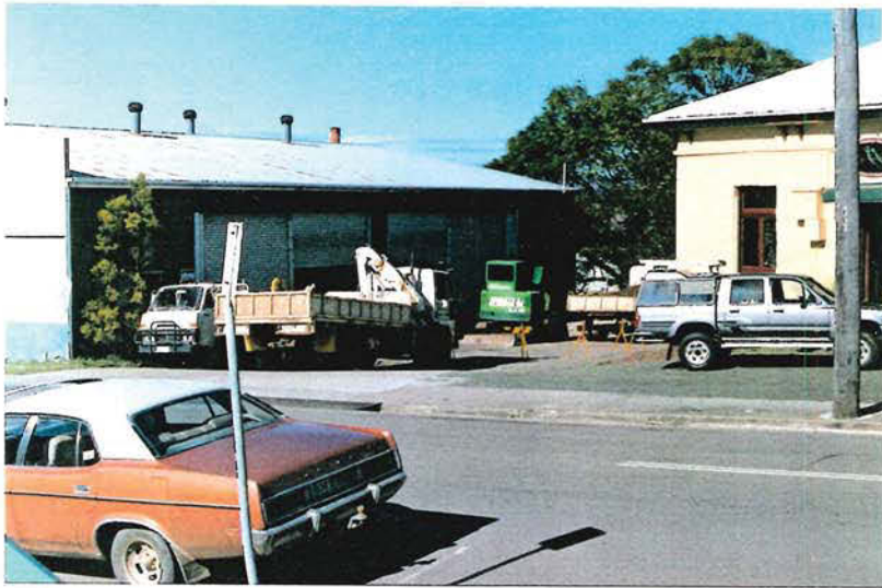
View of site looking south-east across Nash Street. The garage and workshop is on the left side of the photograph.
