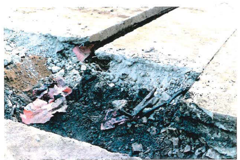
Further excavation of the pump drain area in progress.
