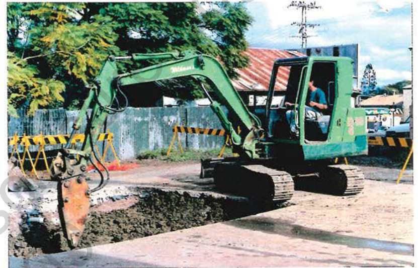
Compaction of the backfill in progress.
