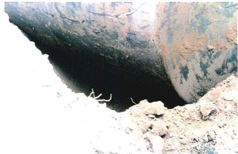
Removal of the tank. Note the dry base of the pit and good condition of the base of the tank.
