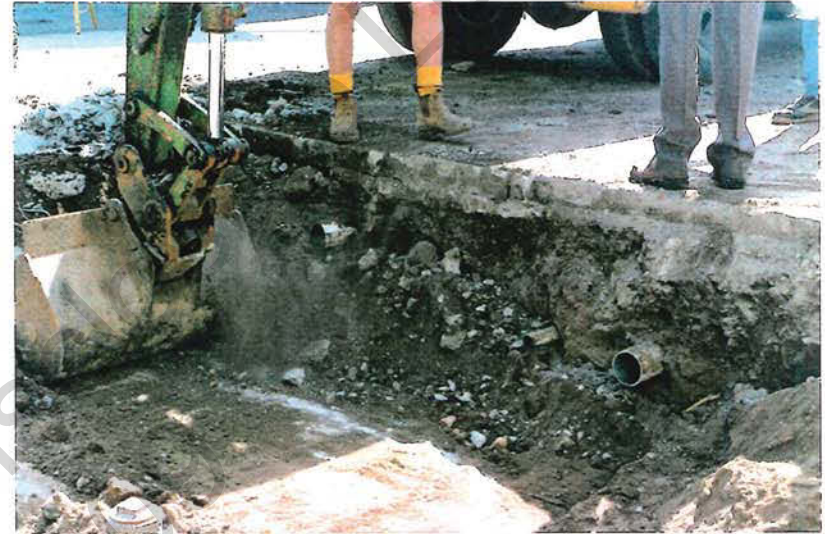
Excavation of the top of the tank. The concrete beneath the excavator bucket is the top of the anchor. Note the two pipes on the right. The pump line is on the left and the fill line on the right.
