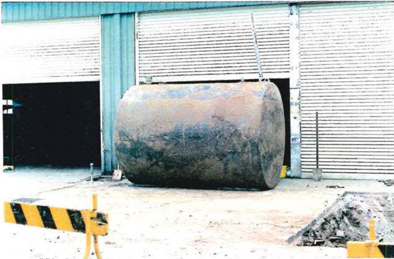
The excavated tank prior to removal from the site.
