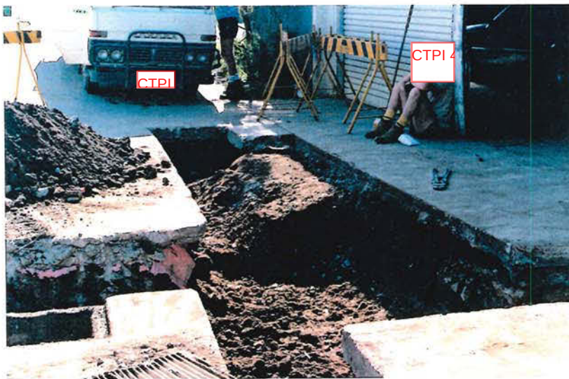
Excavation of the pump drain area completed. View looking north toward the former position of the remote fill point.
