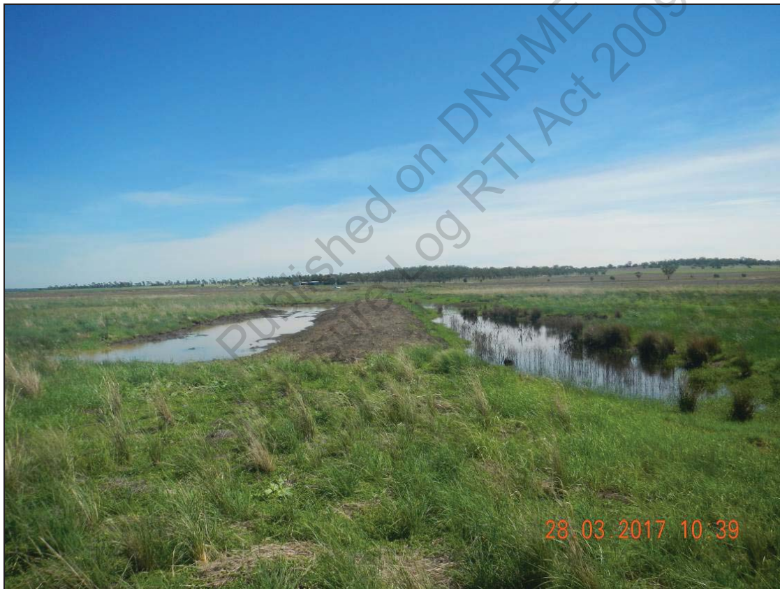
New maintenance work carried out on embankment located on Doctors Creek.
