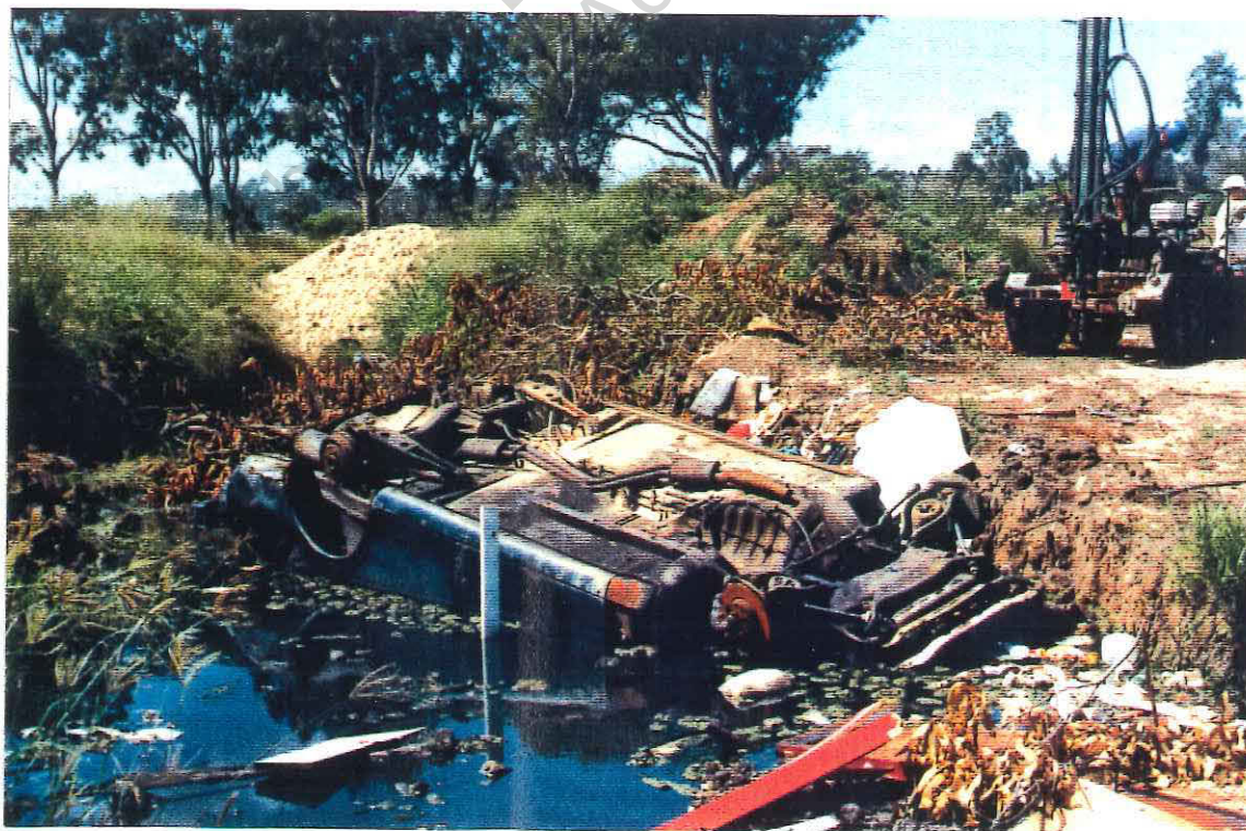
Photograph 15 View to southeast showing another pond at northern end of site used for dumping. Drilling rig for borehole No. 2 on RHS.
