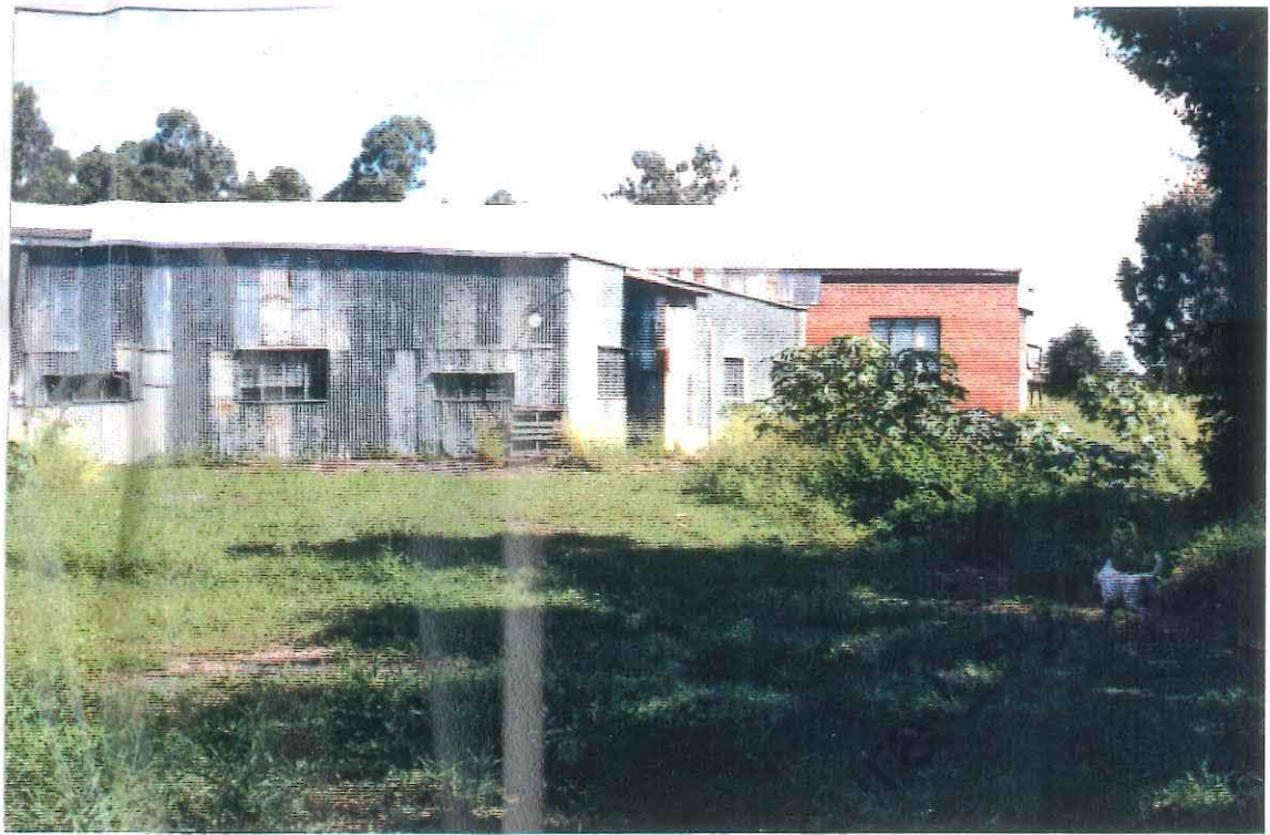
Photograph 12 View to the south at northwest corner of factory, dropping off to the river on RHS. Shed in picture used to be area for chemical storage.
