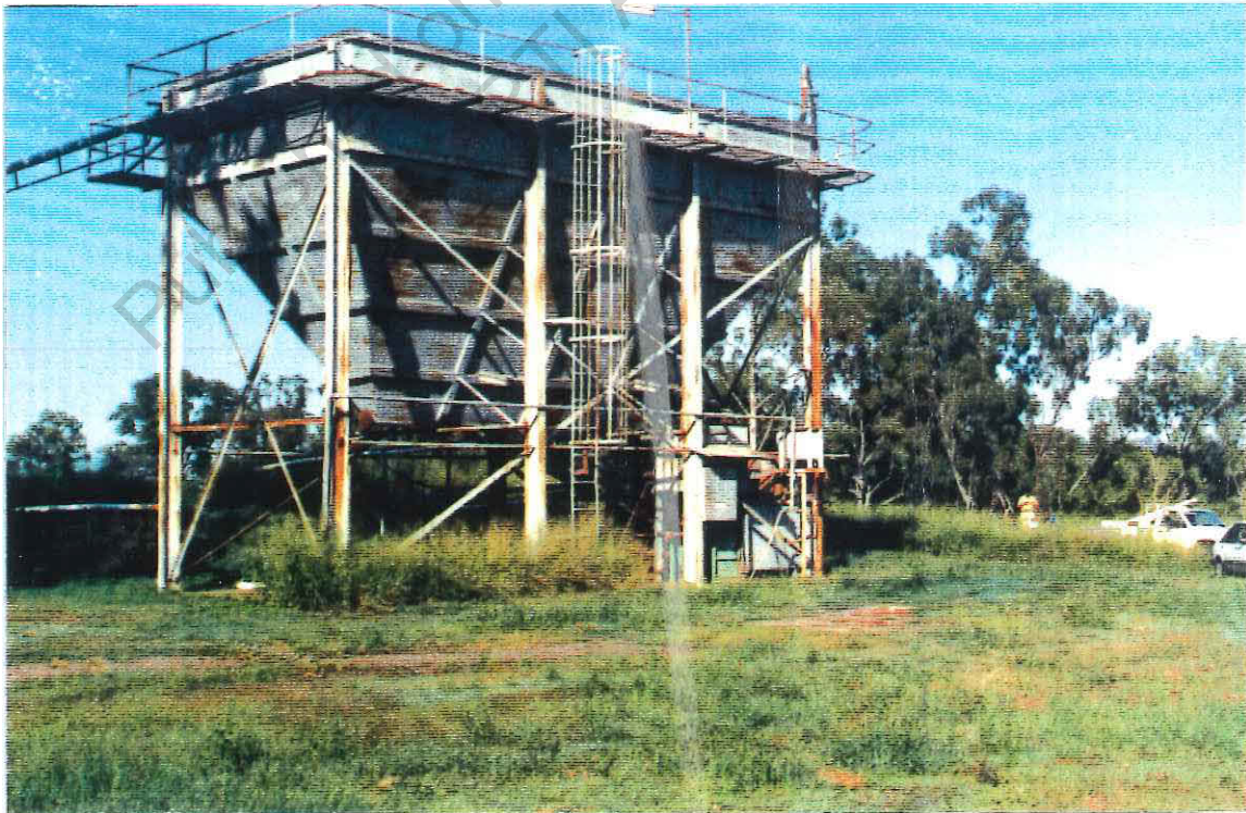
Photograph 5 View to the southwest showing large clarifier at pond 1. (Figure 1). Borehole No. 1 being drilled on RHS.
