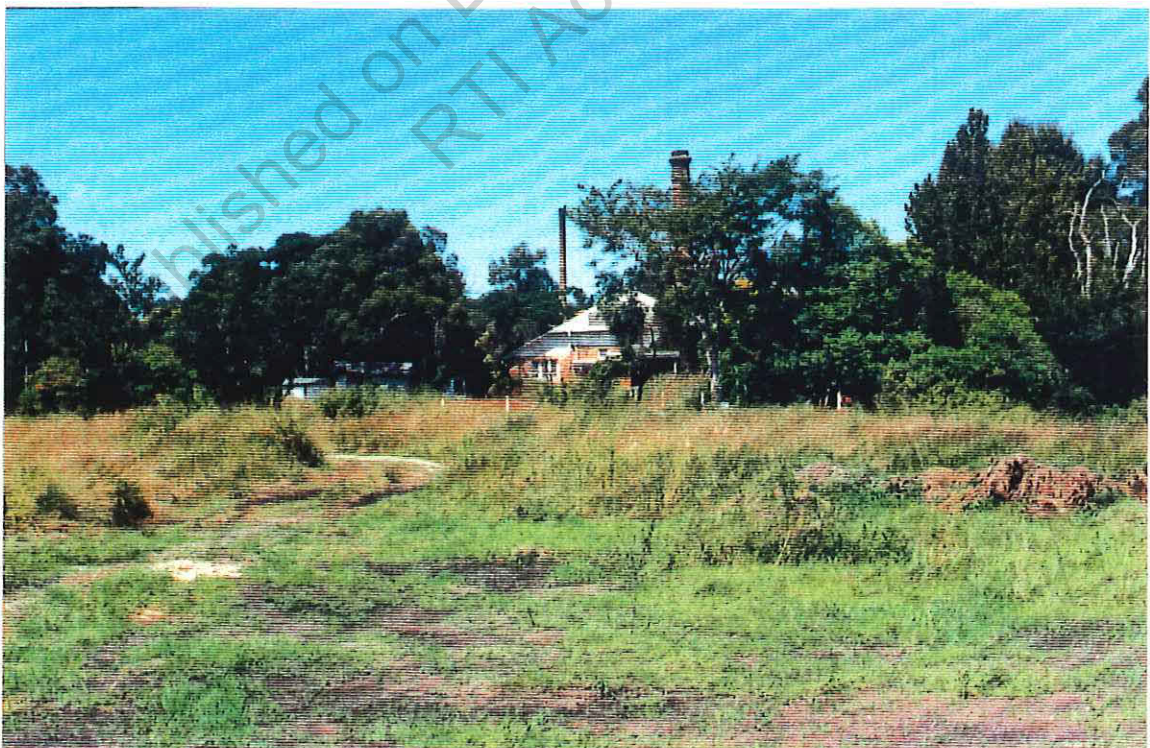
Photograph 11 View to south showing northern aspect of sch4p4(6) Pers dwelling with the smoke stacks of the factory just visible.
