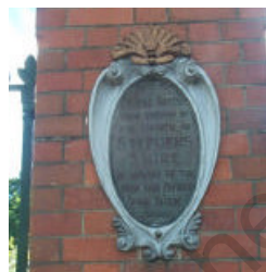
Above: plaque to north pier. Below: plaque to south pier.
