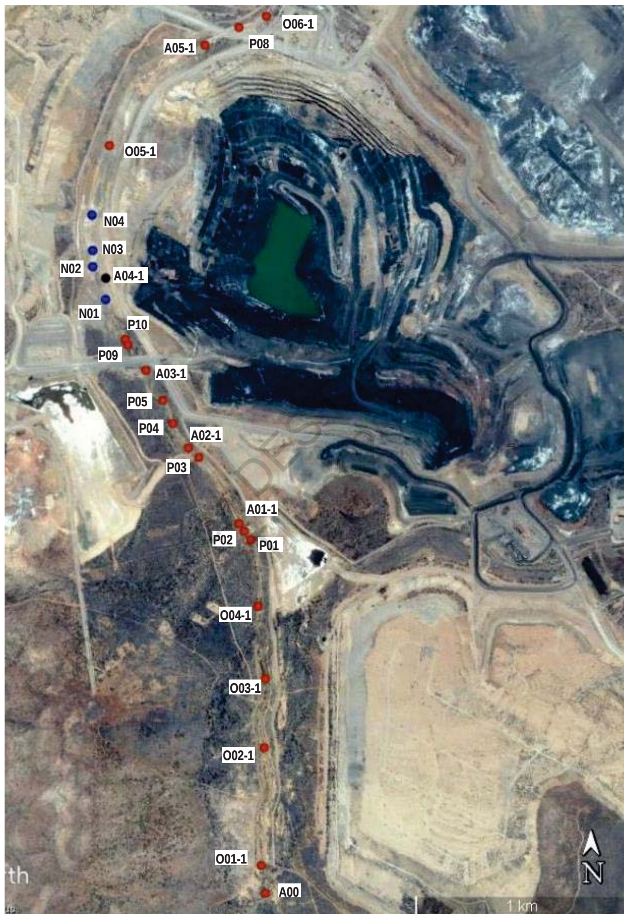
Figure 2.1.3 Page Creek Diversion channel sites sampled in 2014. [Google Earth 2017].
