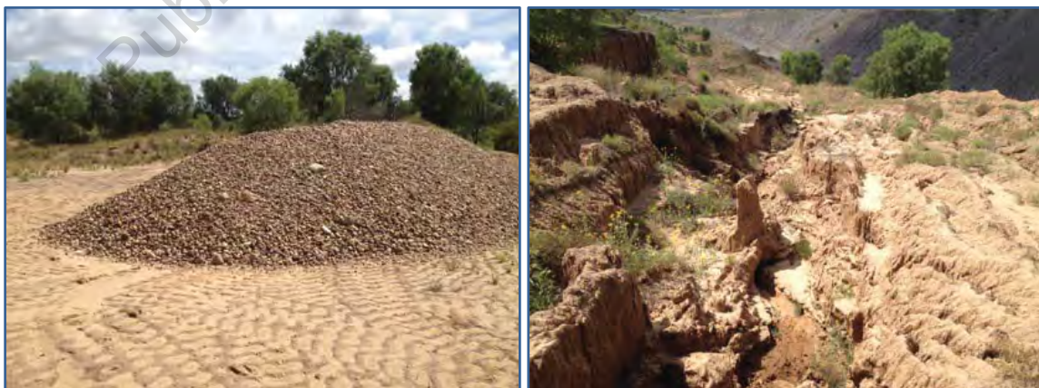
Figure 3-1 Quaternary overburden in B Pit is screened for gravel and sand for use around site (left) and erosion of in situ Quaternary overburden on B Pit endwall (right)
