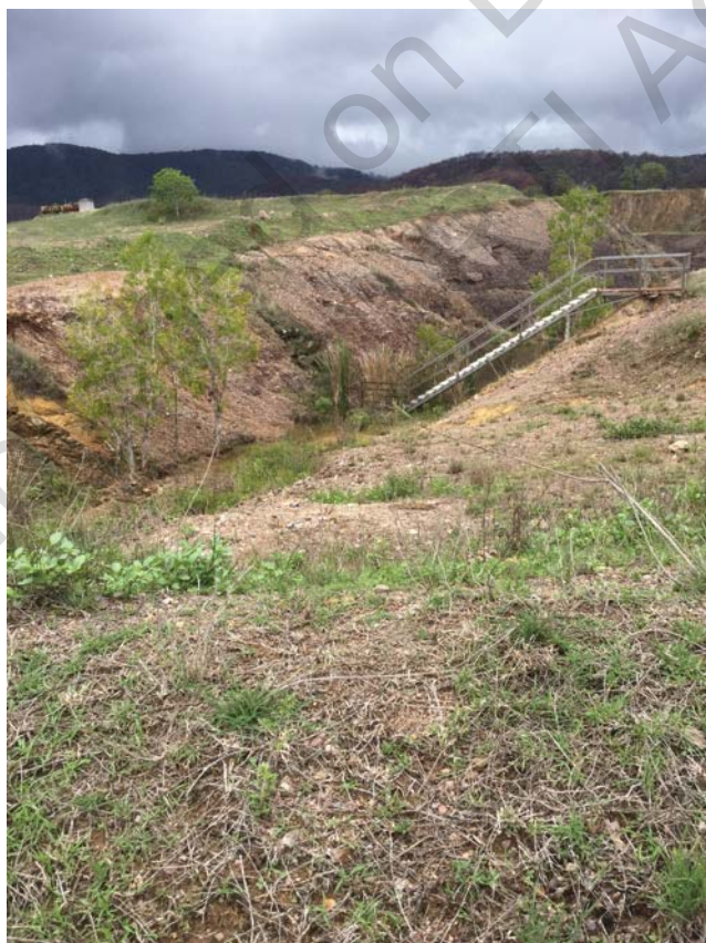
Photo 7: Baillie's Quarry sediment dam
