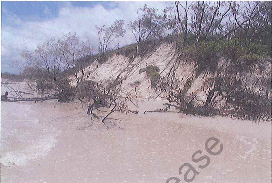
Photo 2: Typical dune erosion along high dunes
