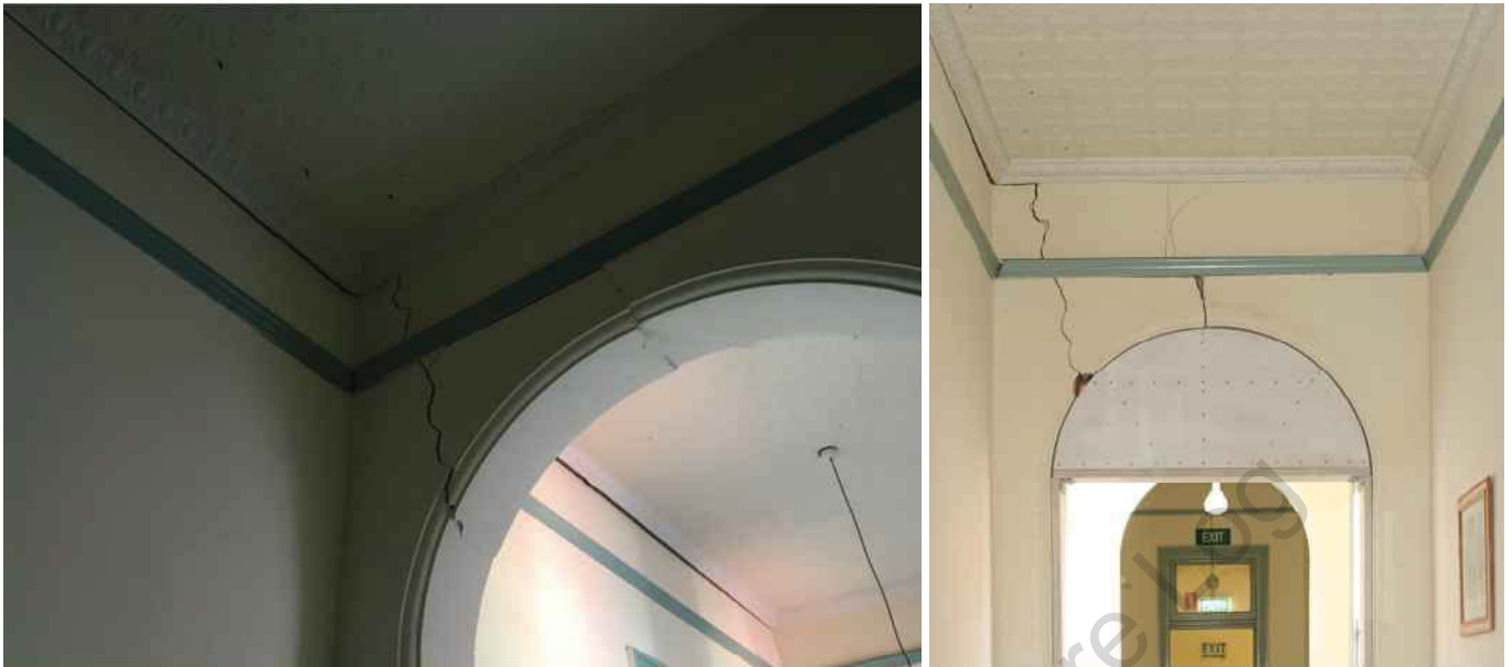
Images 22a (left) an image from the engineers report and 22b (right) the same location with stabilisation works (DES, 23 August 2019).
