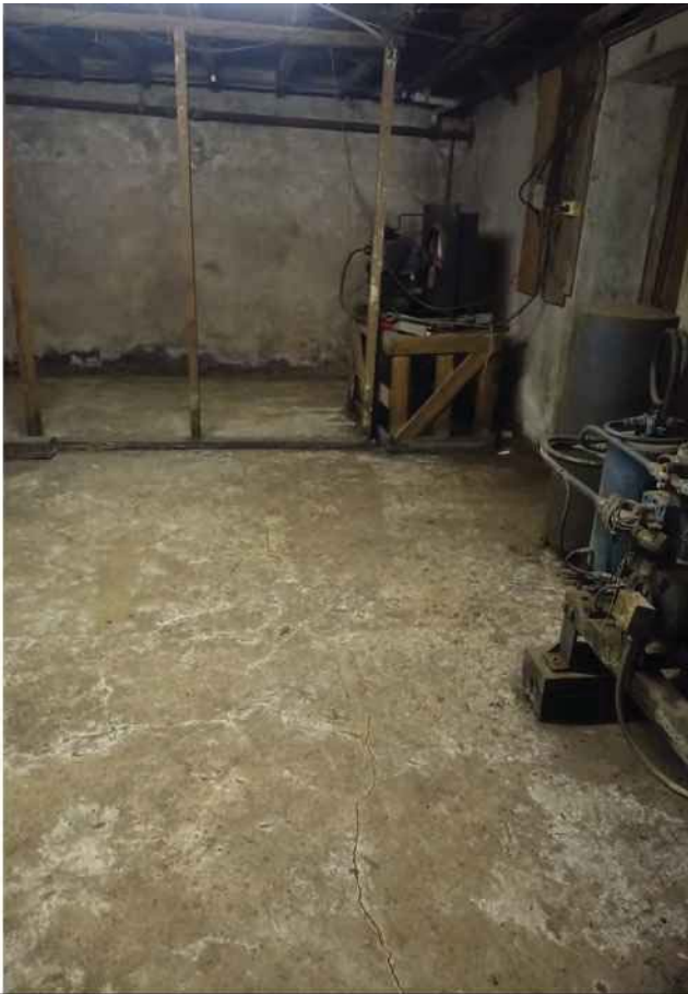
Images 18a (left): Looking across the basement to the northern wall (DES, 23 August 2019). 18b (right) Looking across the basement to the northern wall. Note the alignment of the slab crack relative to the wall cracks. (DES, 23 August 2019.)
