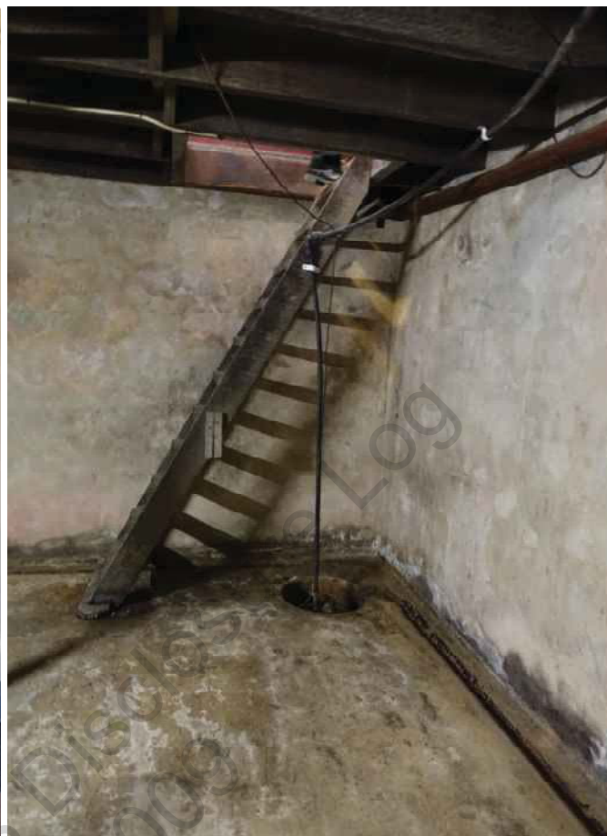
Image 13 (left): The access doors to the hotel's historic cellar in the basement (DES, 23 August 2019). Image 14 (right): the access point and ladder leading from the front north west corner of the public bar. Note the spoon drain and sump in the front right hand corner under the ladder. (DES, 23 August 2019.)
