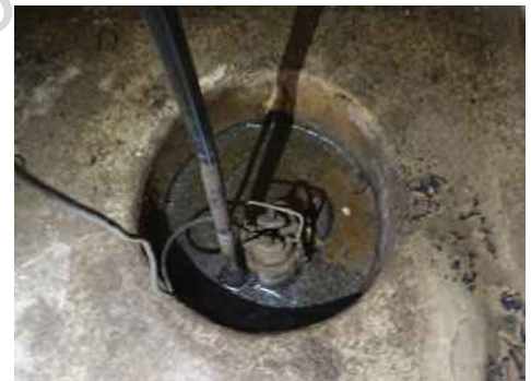
Image 14b (right): The sump with automated pump with water sitting just below surface (DES, 23 August 2019).
