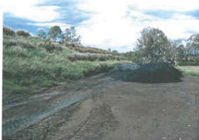
Photograph 11 – Boiler ash bulk storage area below the composting pad (centre left) showing well-established Vetiver Grass bank stabilisation plantings.
