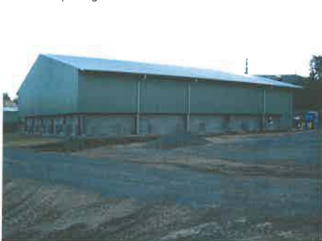
Photograph 12 – Recently constructed bulk hides raw materials storage shed, which has allowed total salted hides storage on site at Josephville, resulting in vacating of the previously long-term rental premises at Redbank.
