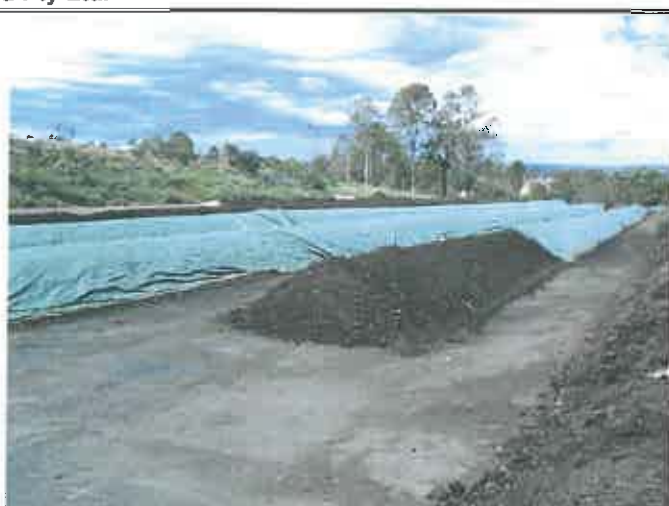
Photograph 10 – Second view of covered and uncovered composting windrows showing the extent of the asphalt sealed mixing/maturing pad.
