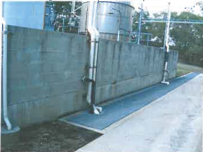
Photograph 14 – View indicating the integrity of a large exposed bund wall servicing a number of separate bays with dedicated liquid storage tanks.
