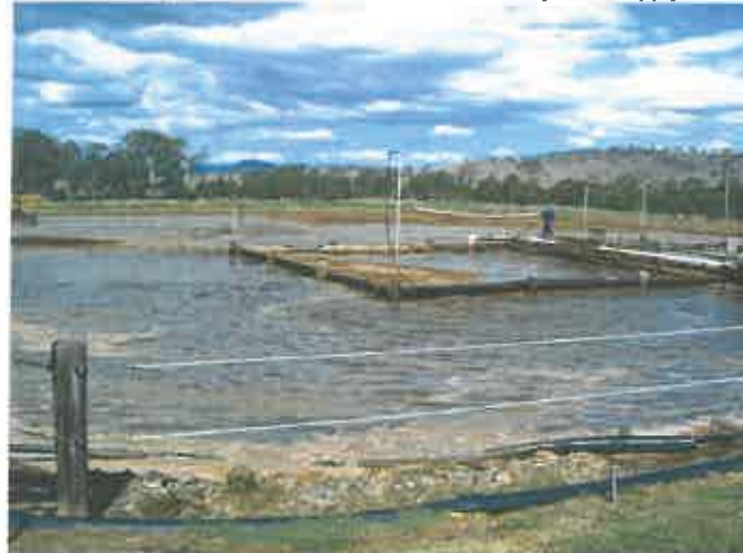
Photograph 19 – Aerobic effluent treatment Pond showing a typically desirable caramel/light chocolate brown colour, together with a very low odour profile noted on the bank of the pond during the site inspection. More effective air mixing/incorporation into the pond contents by way of (6) new Stem-Drive Units has contributed to the real improvements noted in pond operational "health".
