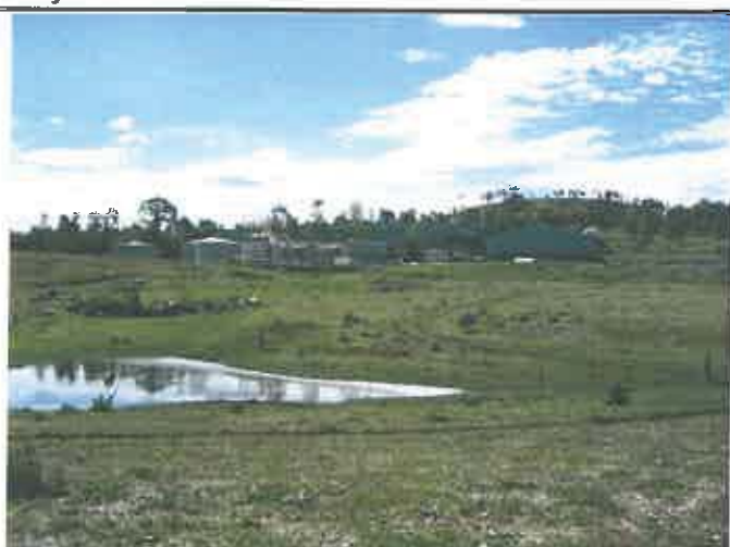
Photograph 4 – Larger "catch" dam of two (2) detention basins (first series dam with rock wall support is on hill above foreground unit) which serve as "first-flush" collectors for the concrete surrounds to the gelatine processing plant (centre skyline). Accumulated material is pump returned to the Aerobic effluent treatment Pond for processing.
