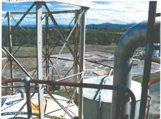
Photograph 22 – Overhead view of the Aerobic effluent treatment Pond showing the desirable caramel/light chocolate brown colour of the "healthy" pond contents.
