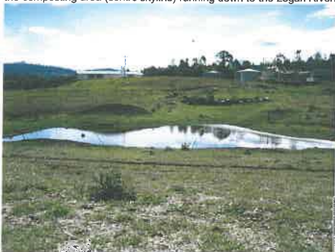
Photograph 6 – Second view of the series pair of "catch" dams which serve as "first-flush" accumulation/holding ponds for drainage from the formed concreted/roadway processing plant surrounds, prior to reprocessing through the Aerobic effluent treatment Pond.
