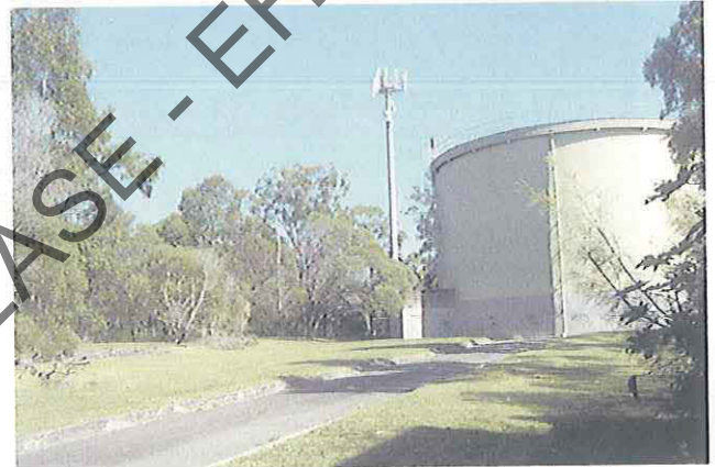
Figure 1.6 – View of the Richlands Water Reservoir and mobile telephone communications tower from Rudyard Street.
