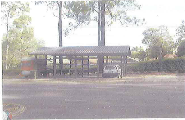
Figure 1.10 – View of the awning within the development site area.
