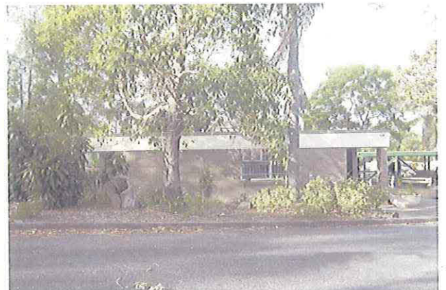
Figure 1.9 – View of the amenity/administration building.
