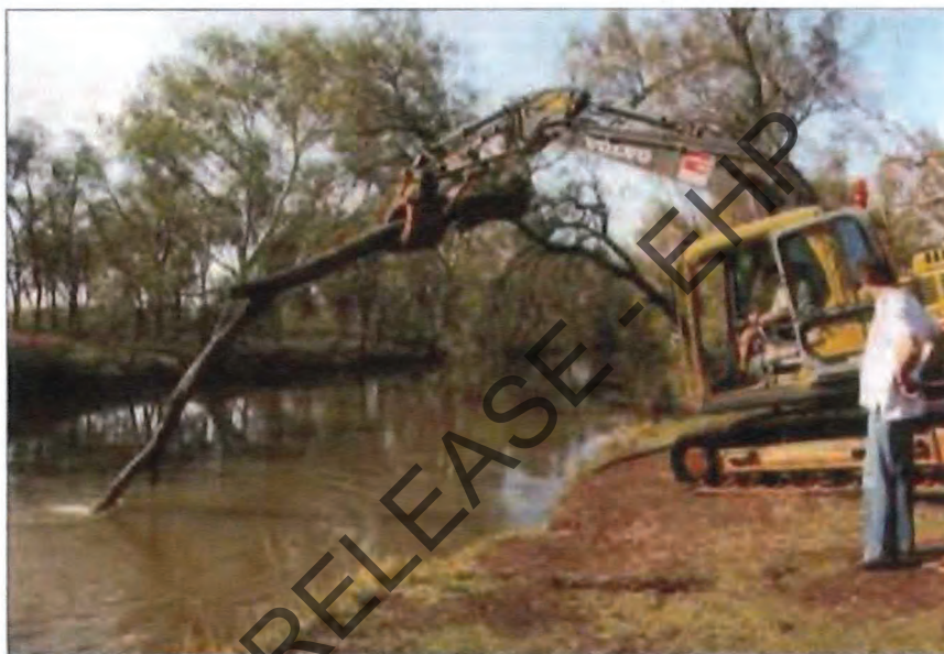
• ABOVE: Mayor Peter Taylor oversees the final logs being placed into Oakey Creek at Bowenville Reserve.
