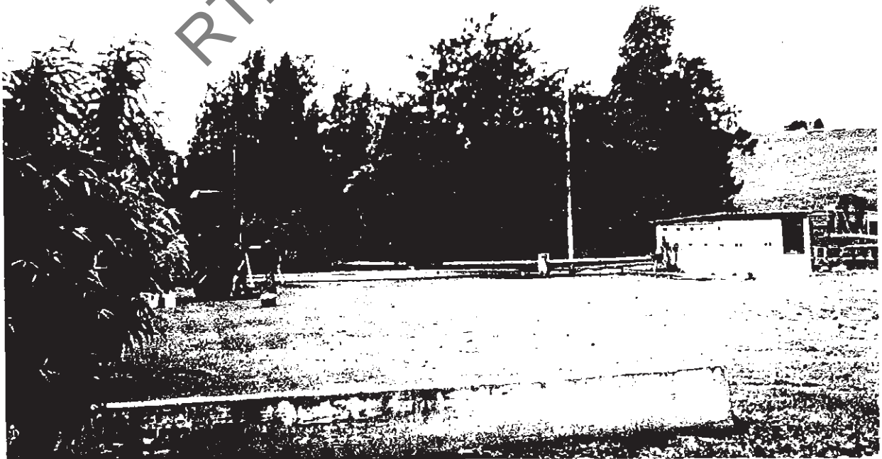
Plate 4: Location of Borehole LB, with the water treatment plant located to the right.
