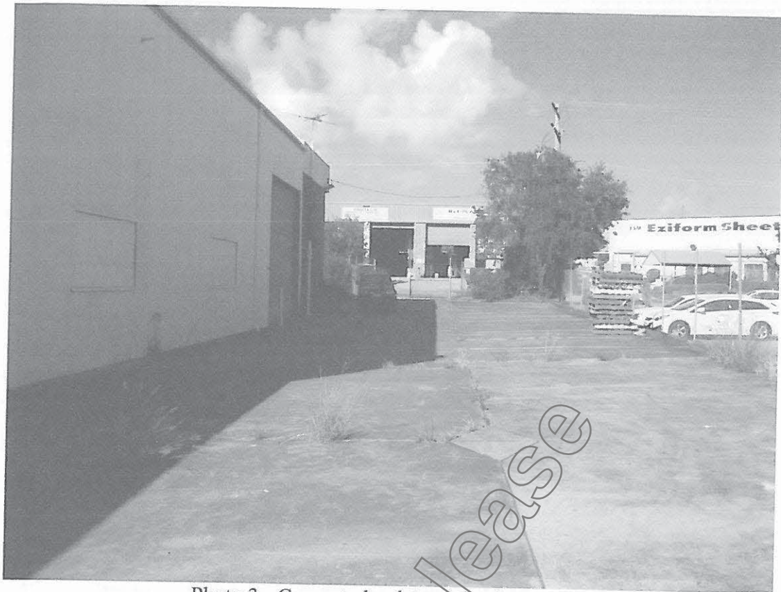
Photo 3 - Concrete hardstand dipping to east
