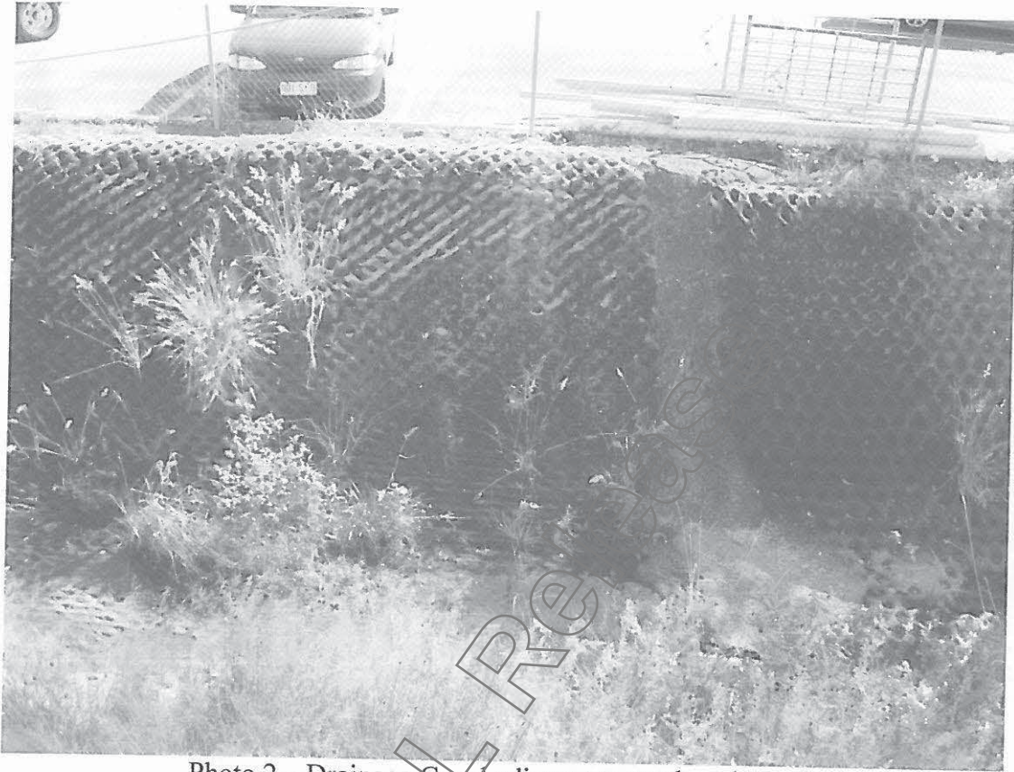
Photo 2 – Drainage Canal adjacent to north end of site
