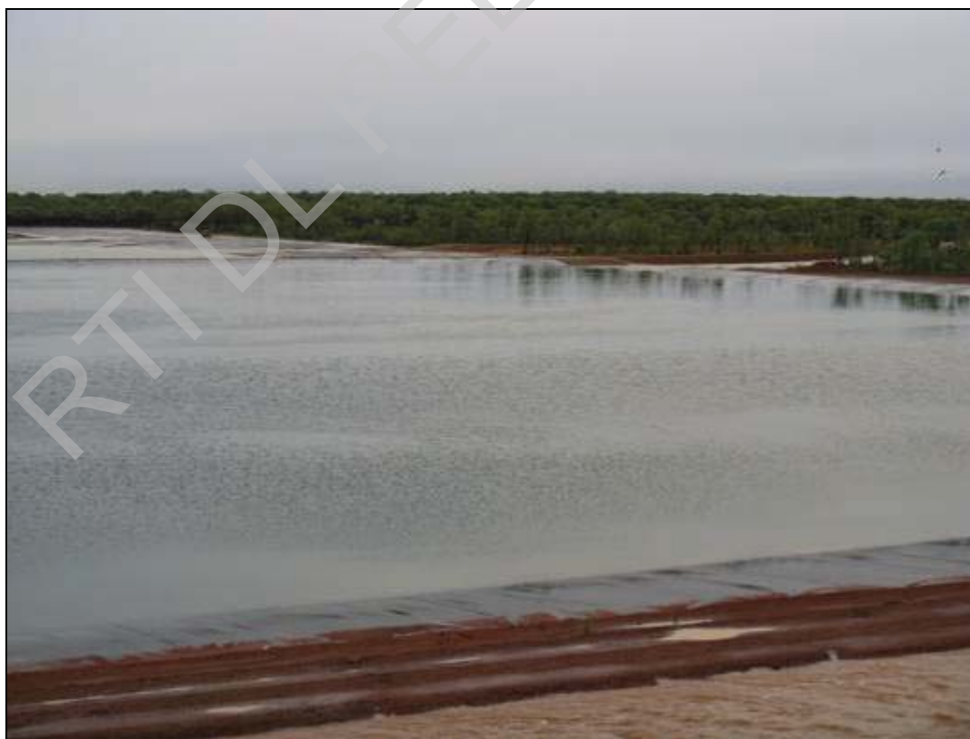
Figure 2: Photo of both Storm Water Pond spillways (Taken 29JAN09).
