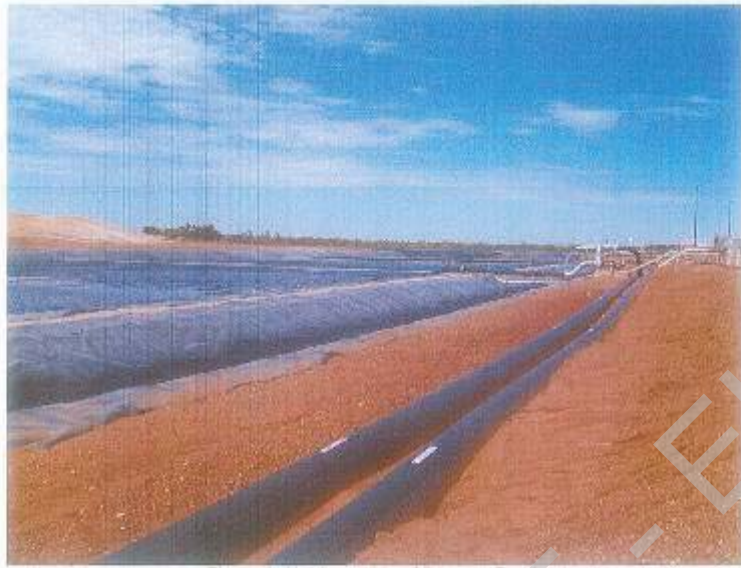
Figure 3: Northern side of Process Ponds
