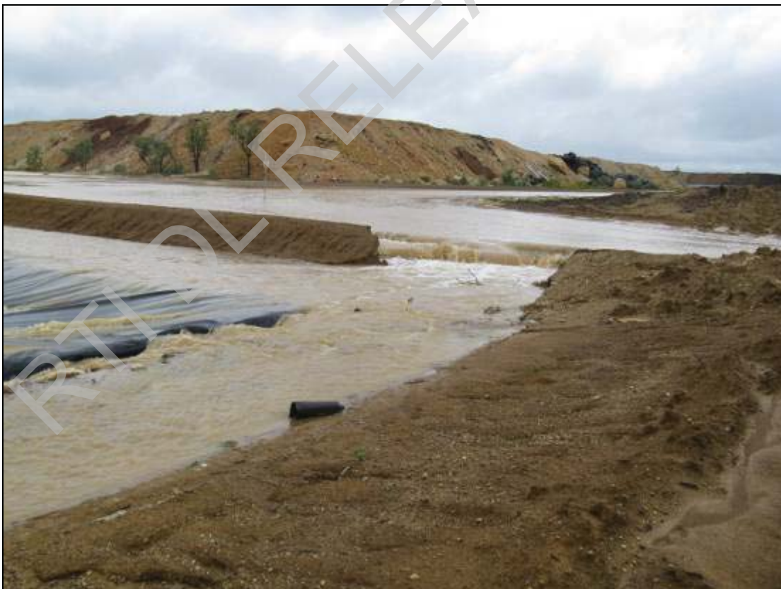
Figure 11: Breach in bund wall on east side of SW Pond #2(Taken 1000 on 30JAN09).
