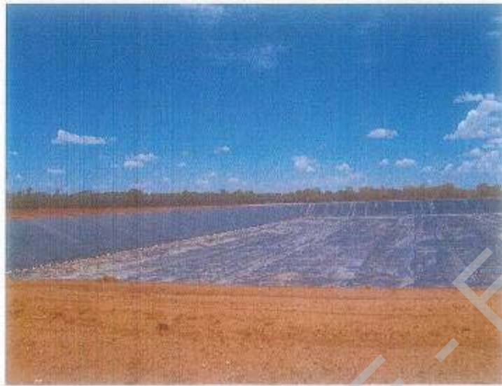
Figure 8: Southern Side of Stormwater Pond No. 2
