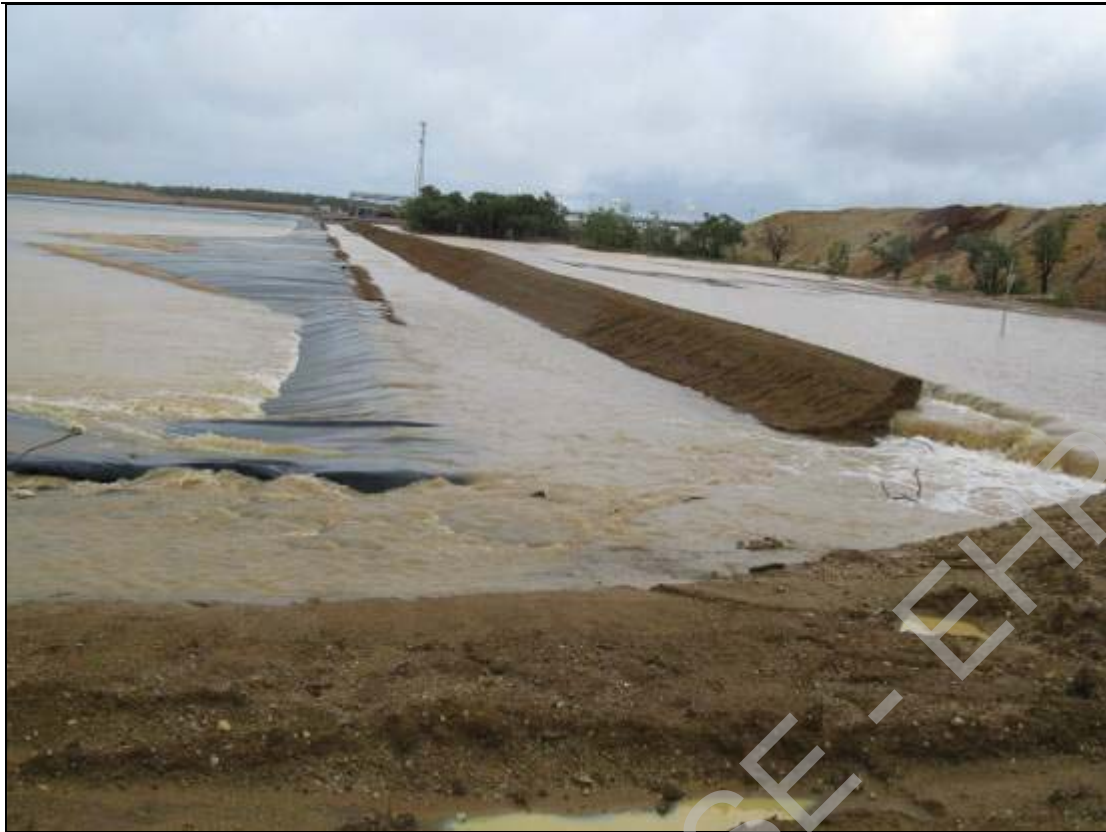
Figure 12: SW Pond #2 looking north towards Processing (Taken 1000 on 30JAN09).
