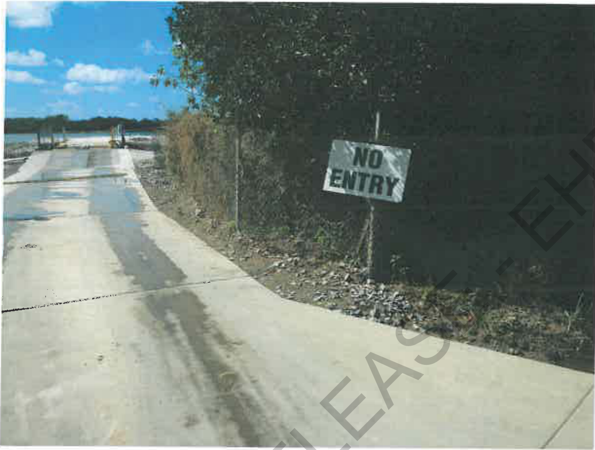
Figure 4 – Signs have been installed directing traffic to enter through one entry and exit out of the other
