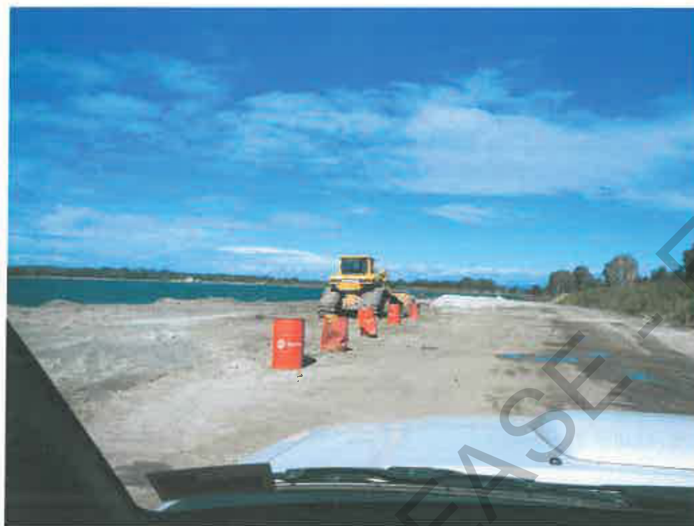
Figure 3 – Pad used for mixing concrete washout and ASS looking South
