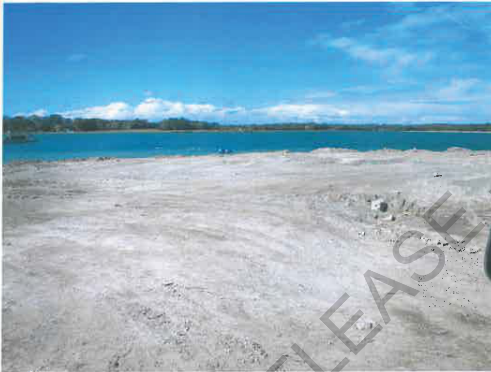
Figure 1 – Pad used for mixing concrete washout and ASS looking South East
