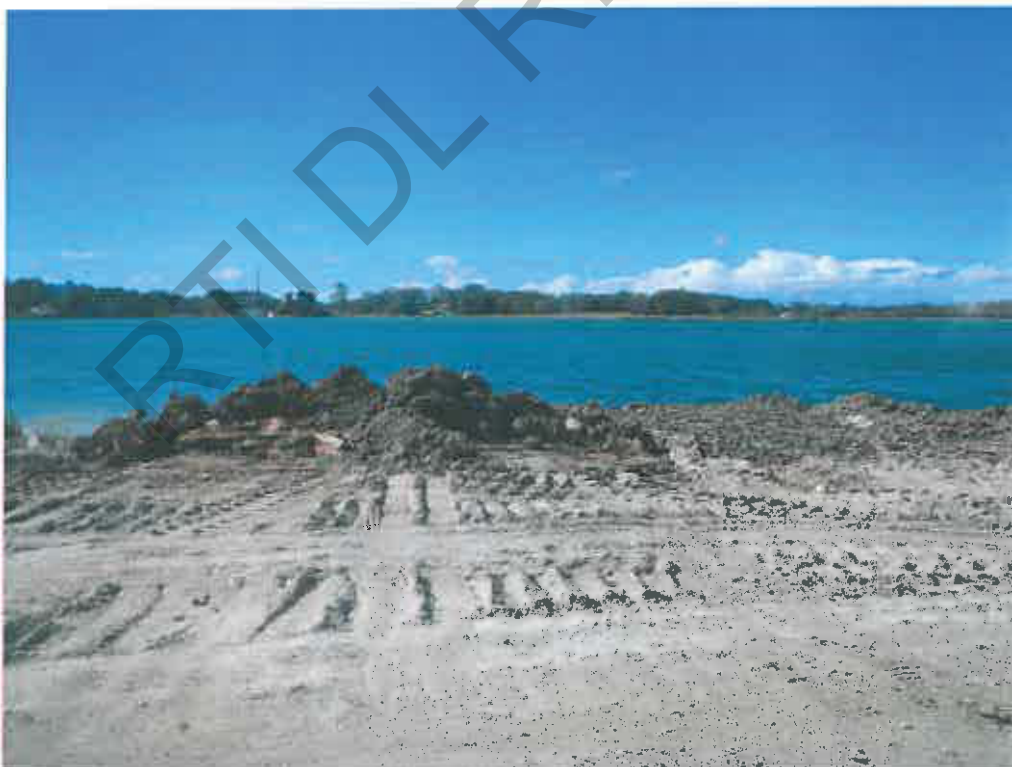
Figure 2 – Pad used for mixing concrete washout and ASS looking East
