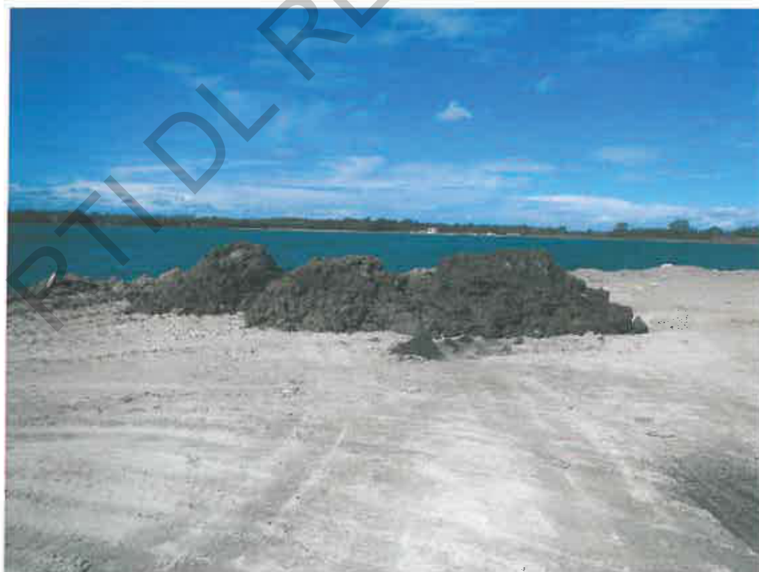
Figure 4 –ASS material on mixing pad
